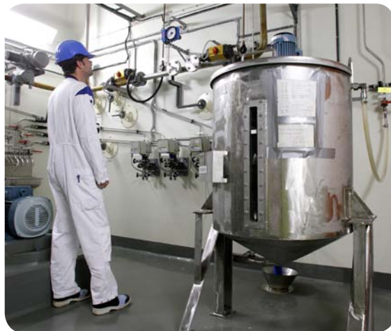
Figure 9-9. Testing and discharge of water Clab.
