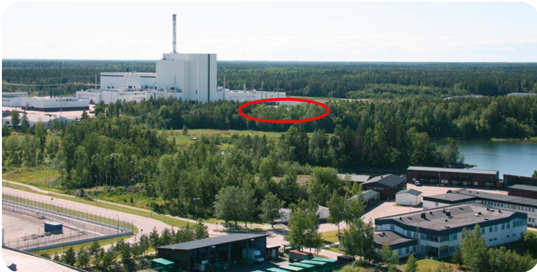
Figure 9-21. Reactor unit 3 in Forsmark, where the red oval shows the area considered for a siting of the encapsulation plant.
