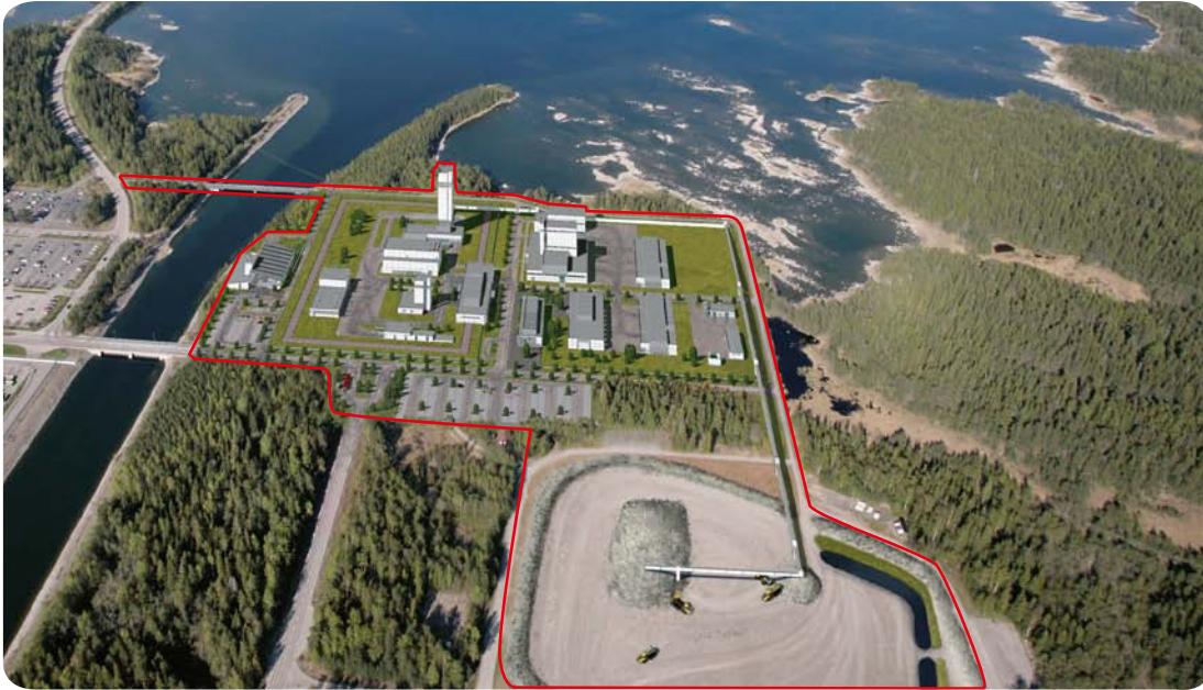
Figure S-7. Location of the final repository on Söderviken in Forsmark (photomontage). The Forsmark Nuclear Power Plant can be seen to the left in the picture, and the area at the bottom is the rock heap. The red outline indicates the part of the picture that is a photomontage.
