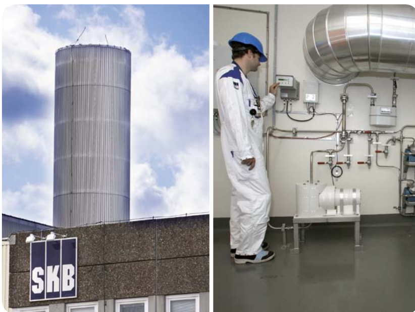
Figure 8-15. Clab's ventilation chimney and measurement equipment for radioactive releases to air.
