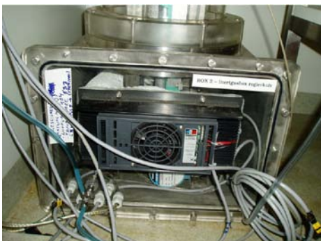
Figure 2-5. Inert gas box for the pressure regulator piston. The pressure regulator consists of a step motor (lower picture) which operates a piston in a PEEK mantled cylinder (upper picture). The motor is controlled by a separate electronic unit. The desired difference pressure between the test section (KA3065A03:1) and the reference section (guard section KA3065A03:2) is set using the control unit.
