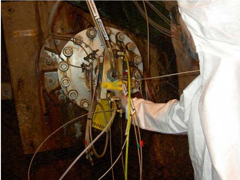
Figure 3-3. The yellow coloured Epoxy resin being injected at the borehole collar.
