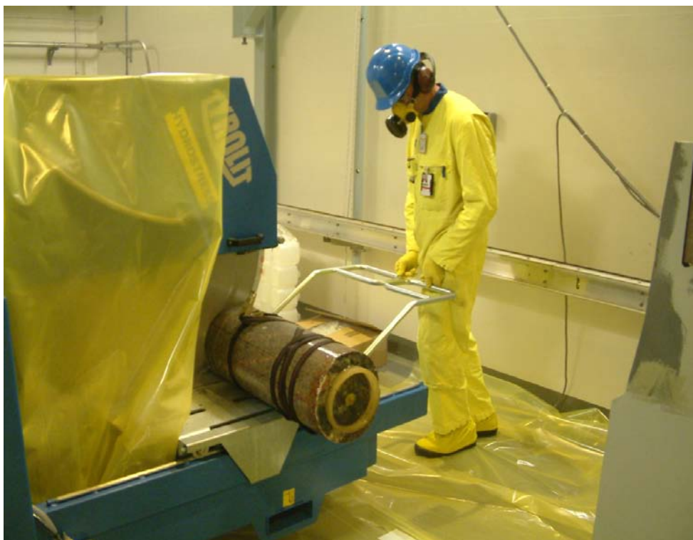
Figure 2-3. Cutting of the core.
