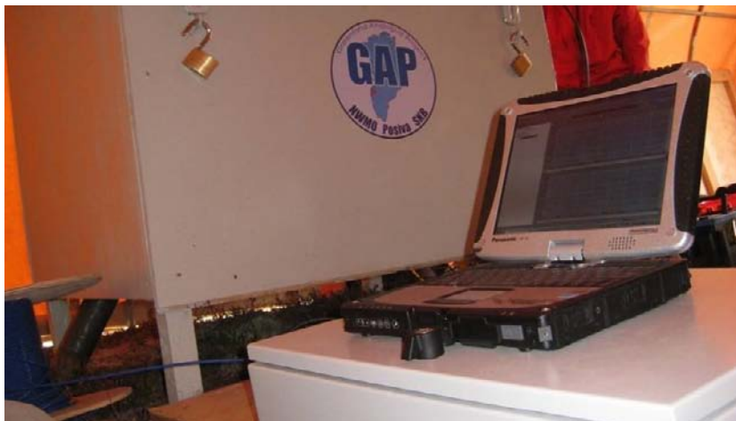
Figure 4-31. Ongoing DTS-measurement at borehole DH-GAP01. The DTS-device is located under the Toughbook computer. Photo by Jon Engström.
