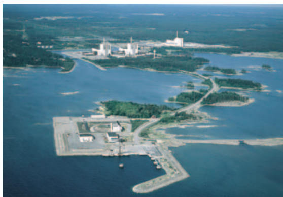
Aerial view of the surface part
