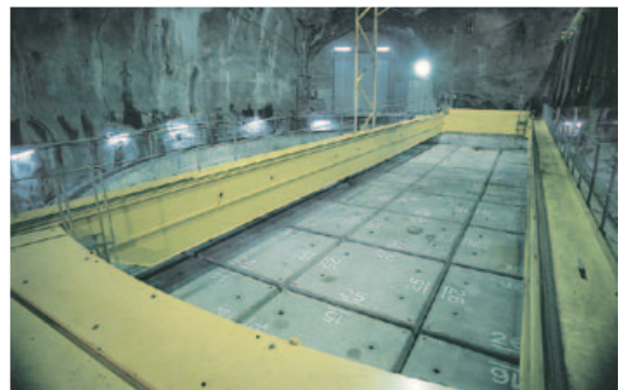
View over top of silo
