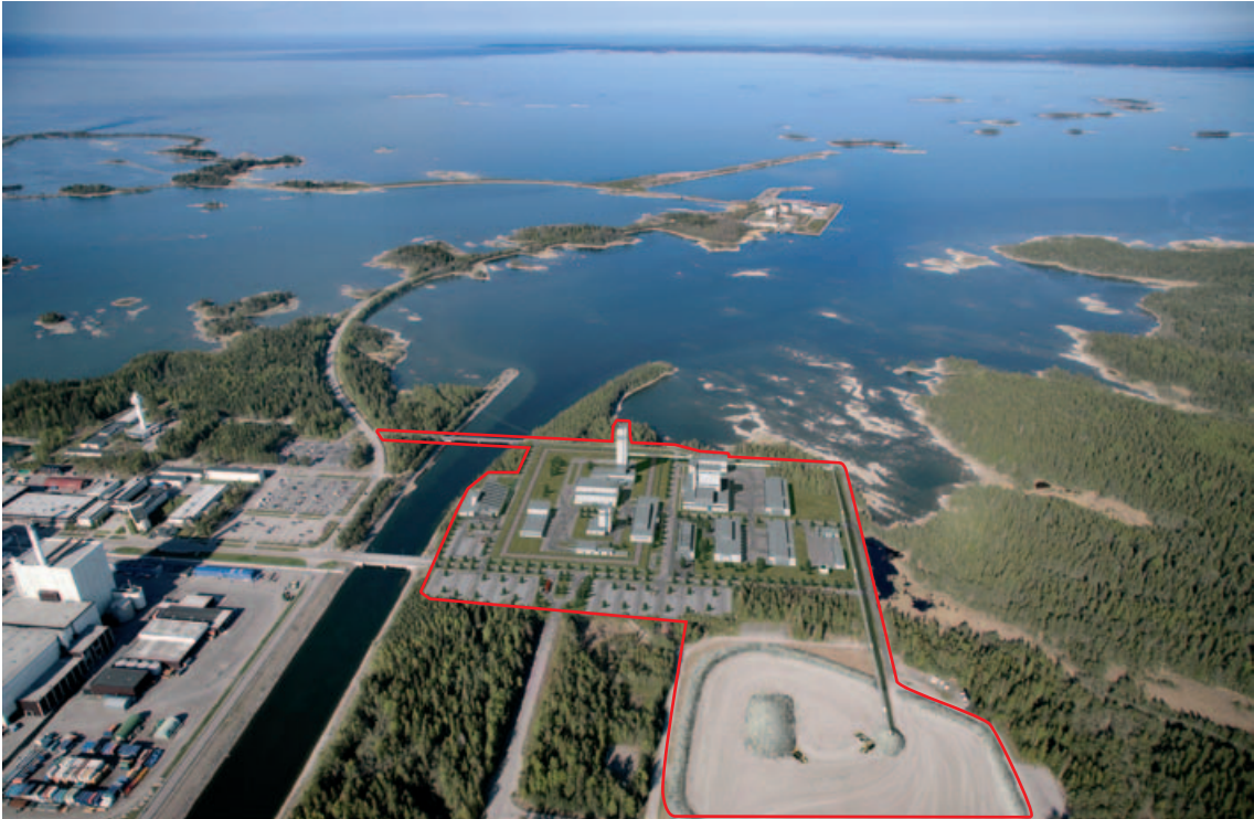
Figure 8-4. Photomontage with the above-ground parts of the planned final repository in Forsmark. The red outlines show the operations area and the heap for rock spoils. Parts of the nuclear power plant can be seen at the left.
