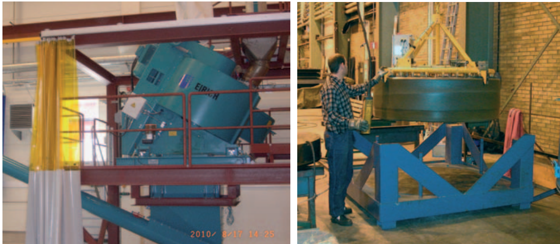
Figure 12-2. At left: Eirich mixer used for conditioning of bentonite at the Äspö HRL. At right: A bentonite block is placed on a shipping pallet.
