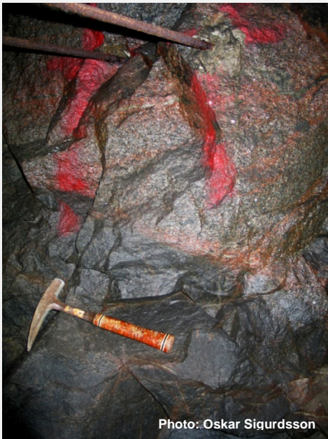
The Tasa-tunnel, right wall, section 46-47 m. Boundary between the rock types Fine grained dioritoid (lower part) and Ävrö granodiorite (upper part.). Geological map of the tunnel face (right).
