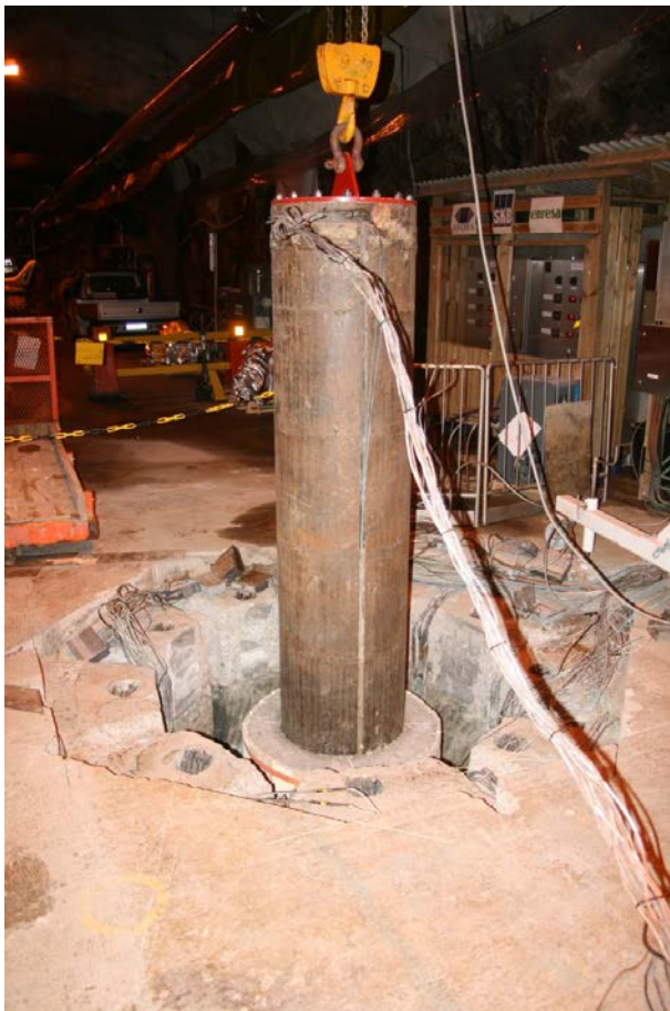
Figure 4-1. The lifting of the lower heater in the excavation of the Temperature Buffer Test.
