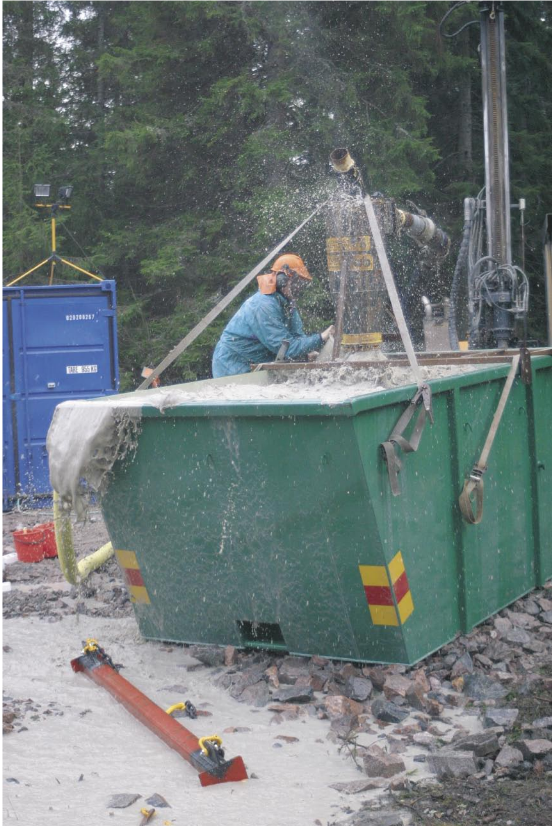
Figure 5-4. Discharged groundwater (c 1800 L/min) during drilling of borehole HFM16.
