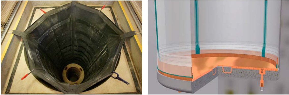
Figure 5-12. The protection sheet installed in a deposition hole. The sheet is attached to the border of the copper plate in the bottom of the deposition hole.
