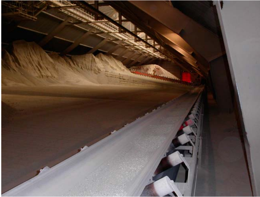
Figure 5-4. Store with scraper for automatic discharge (Minelco AB, Luleå).
