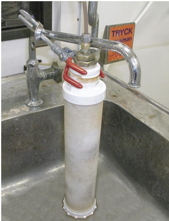
Figure 4-3. The ion exchange column mounted to the outlet of pumped groundwater from the borehole section.
