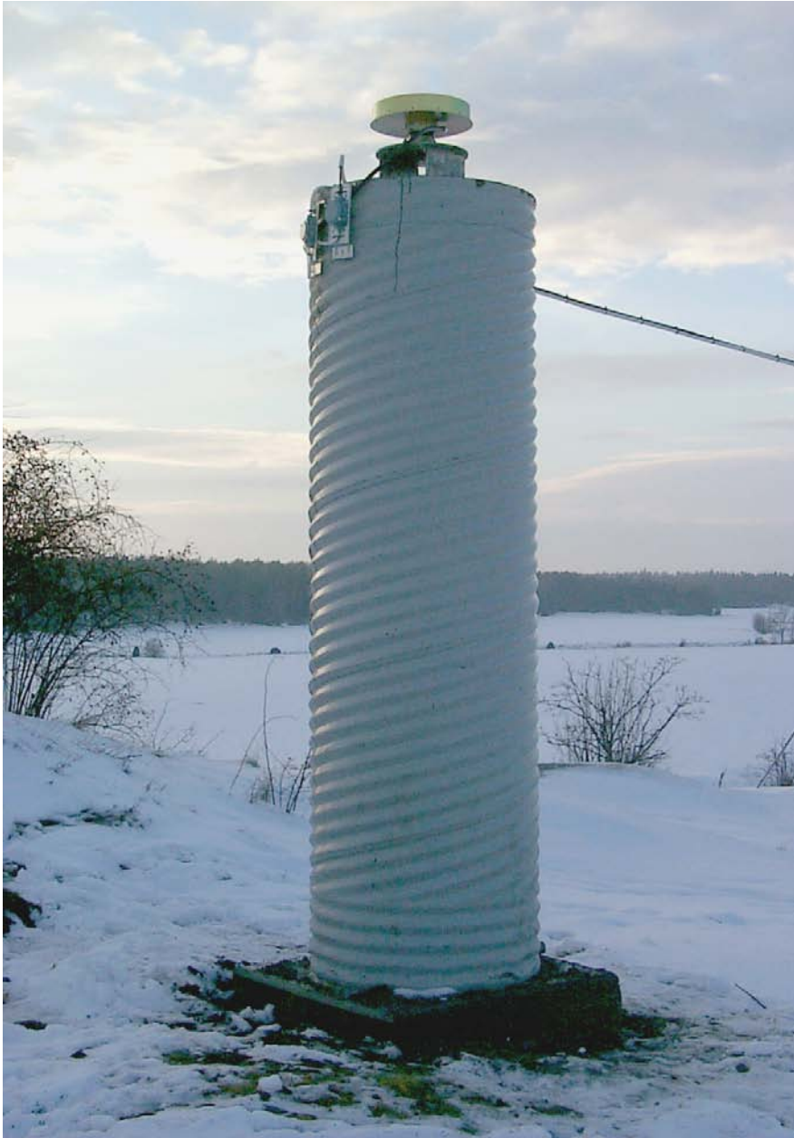
Figure 4-1. The SWEPOS reference station in Uppsala.
