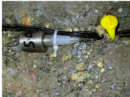
Figure 2-10: Cable and electrode fixation in the backfill
