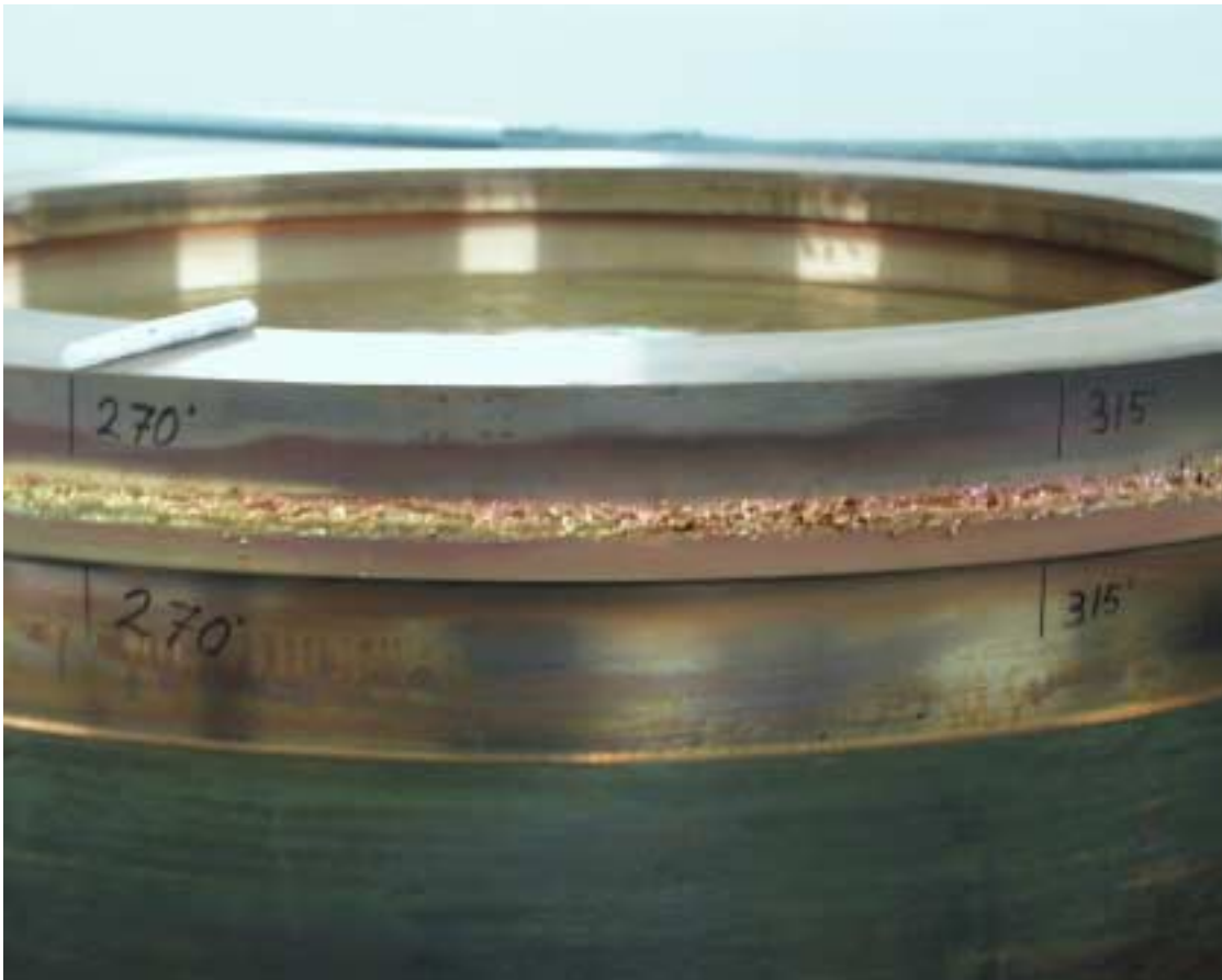
Figure 21: Lid weld no 21, view of the weld surface.
