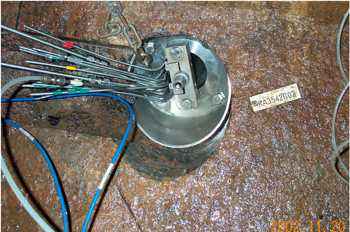
Figure 2-15 Borehole enlargement in the tunnel floor with anchorage for borehole equipment.
