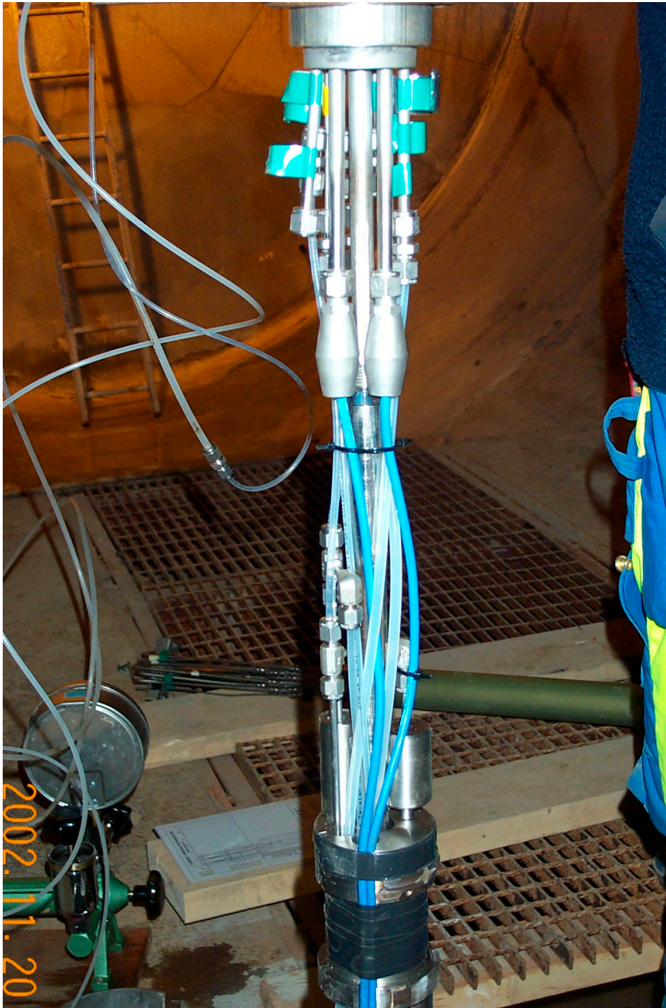
Figure 2-12 Installing HM equipment. Tubes and connections between upper anchor and packer.
