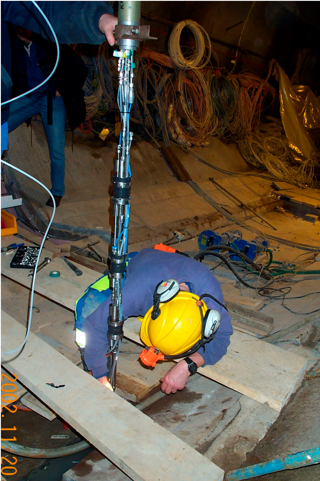
Figure 2-11 Installing HM equipment.
