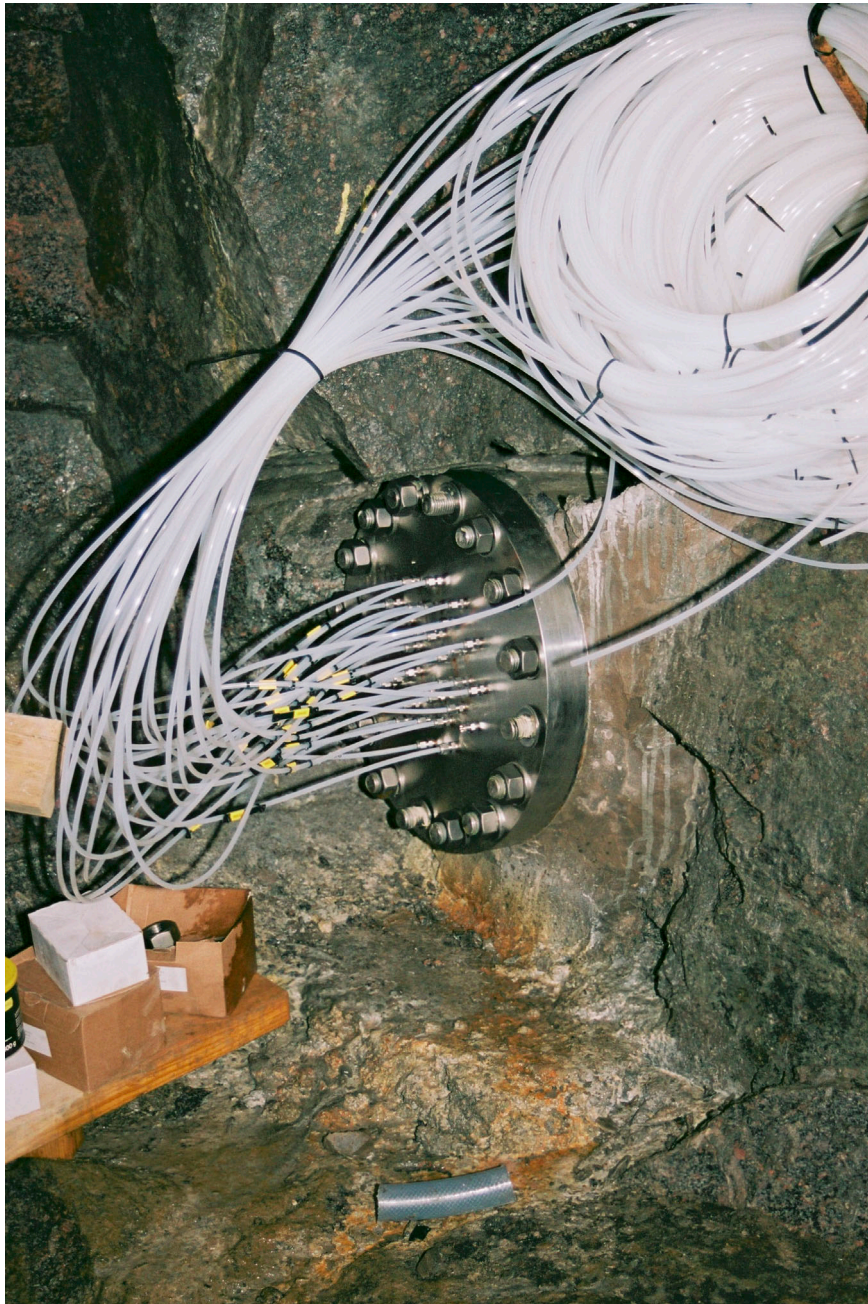
Figure 2-27 Lead-through holes with lid fixed.
