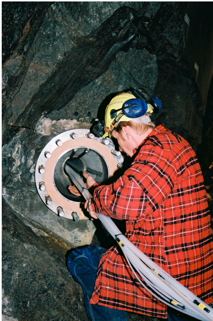
Figure 2-25 Tubes and cables being installed in a lead-through hole.
