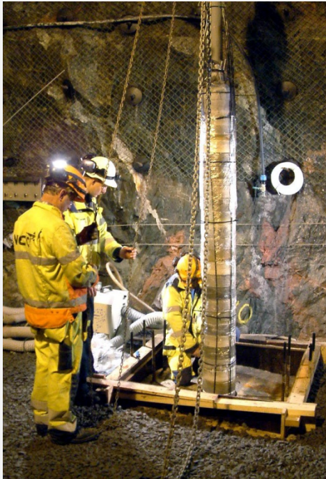
Installation of one of the three test parcels. The photo illustrates the mixing of different compacted buffer blocks.
