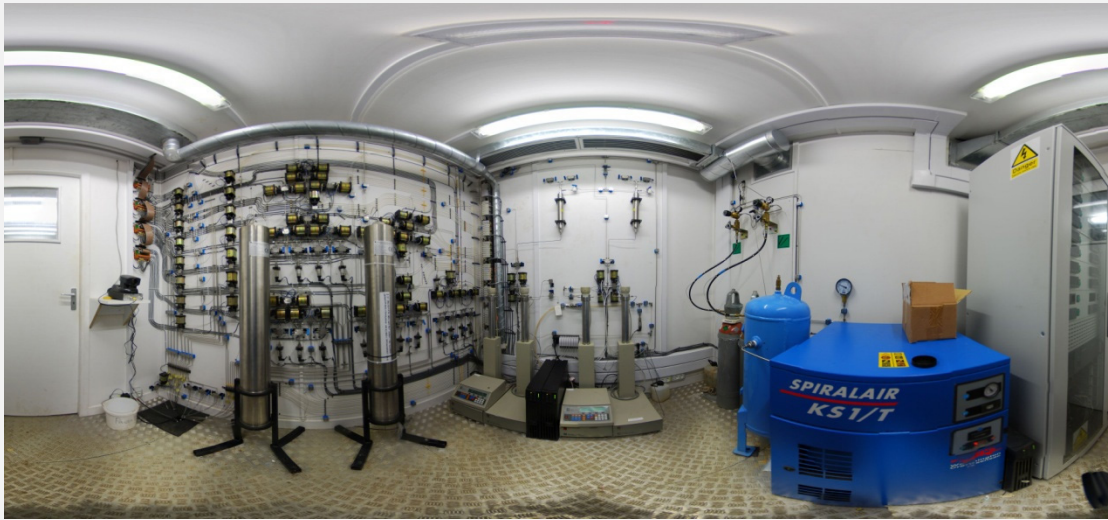
Panorama of the laboratory of the Large-scale gas injection test (Lasgit) at -420 m level in Äspö HRL.
