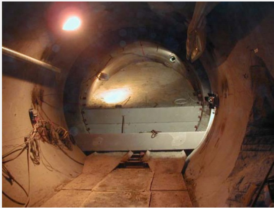
The plug installation for section I in the Prototype Repository
