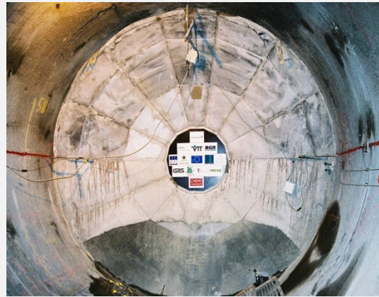
The plug installation for section I in the Prototype Repository
