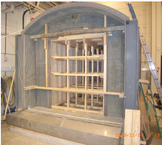
Preparation of Test 4 in the half-scale steel tunnel.
