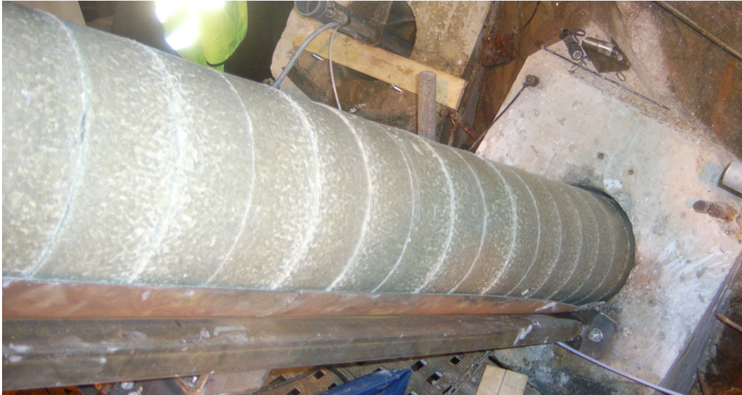
Figure 4-4. Installation of clay blocks.
