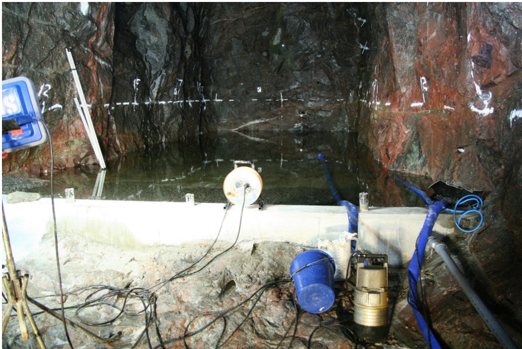
Figure 4-1. Water filled measuring weir in the project Sealing of Tunnel at Great Depth.
