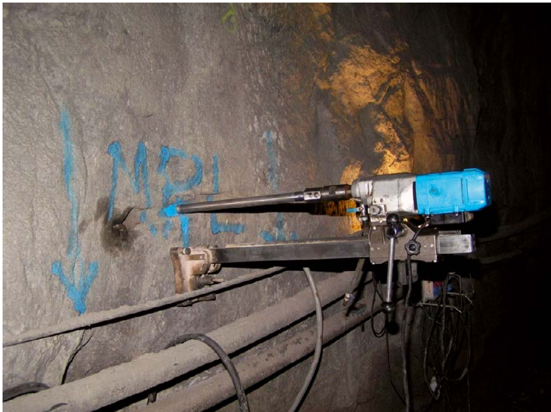
Figure 6-1. Drilling, diameter 32 mm, for the purpose of single-hole testing.
