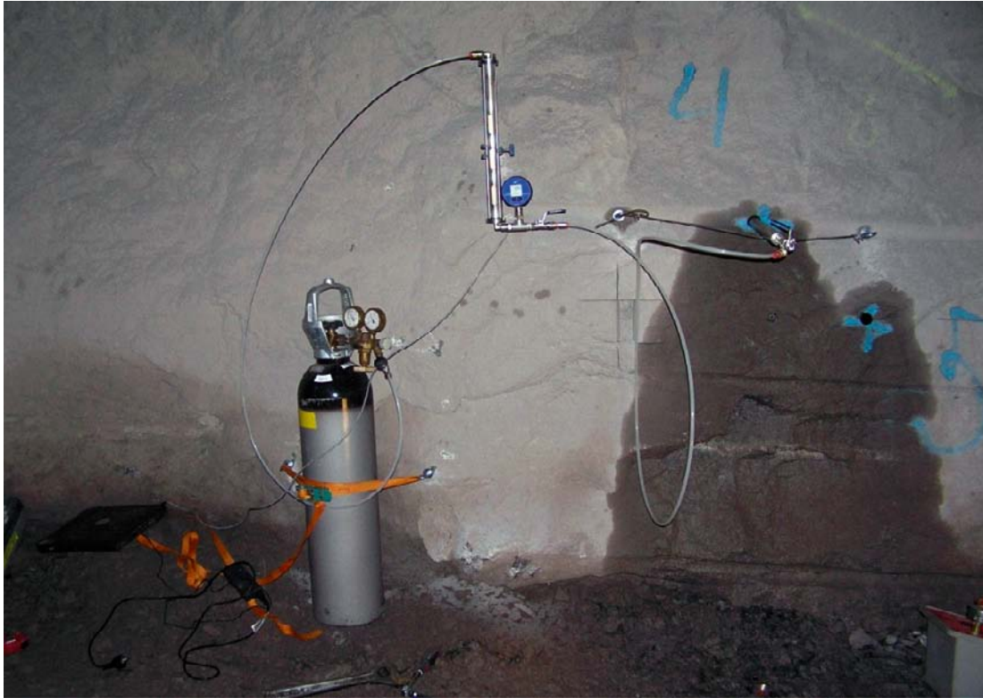
Figure 6-2. Equipment for single-hole testing.
