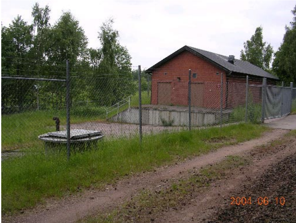
Field observation point 23, photo d. Direction west.
