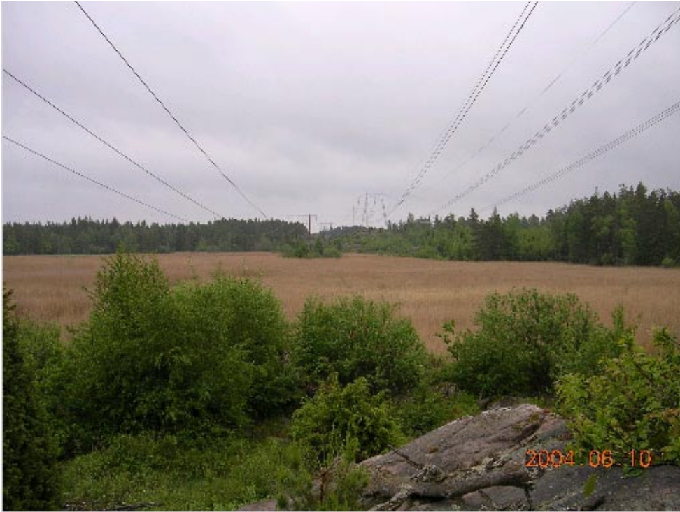
Field observation point 5, photo c. Direction southeast
