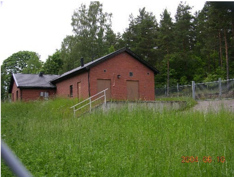
Field observation point 23, photo c. Direction north.
