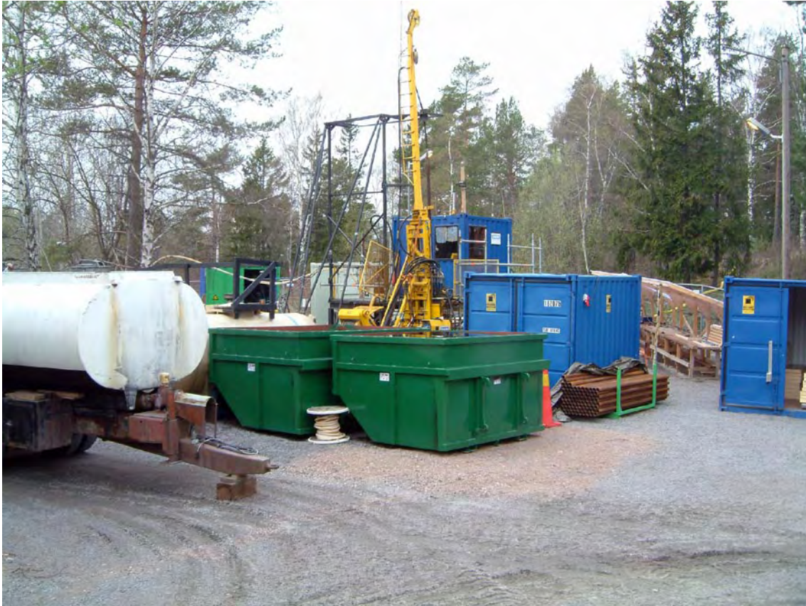
Figure 4-1. The KSH02 drill site.
