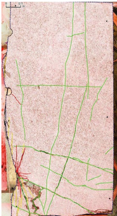
Figure 7-1. Example of a section with a lot of blasting fractures at the lowest hole and hardly any at the two upper holes. Section 40B-03.
