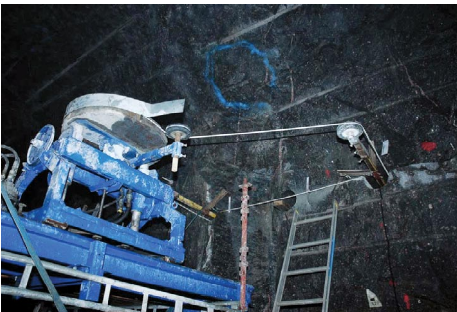
Figure 4-5. Wire sawing of a horizontal cut.
