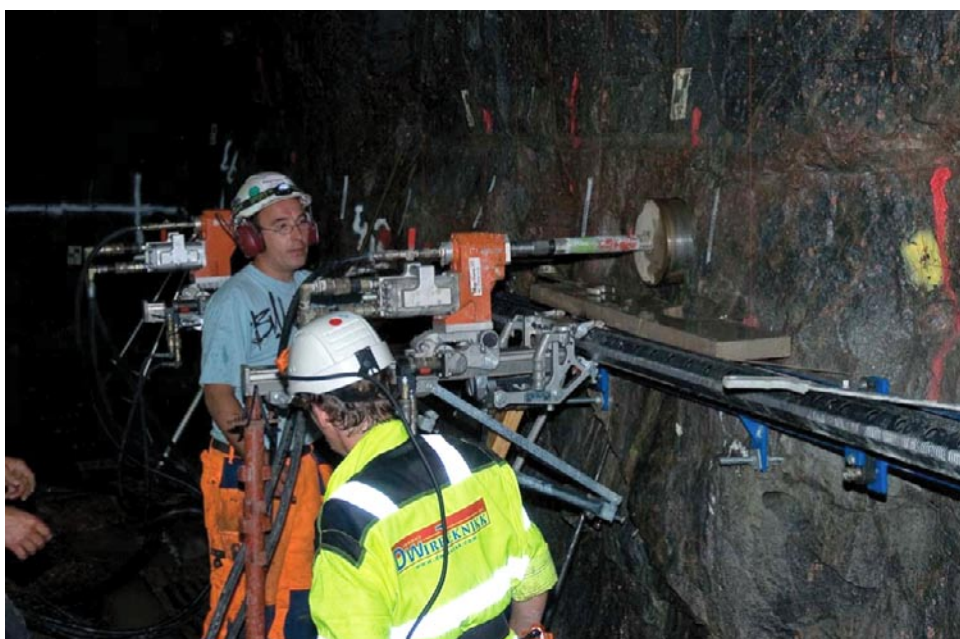
Figure 4-3. Core drilling of wire sawing holes.
