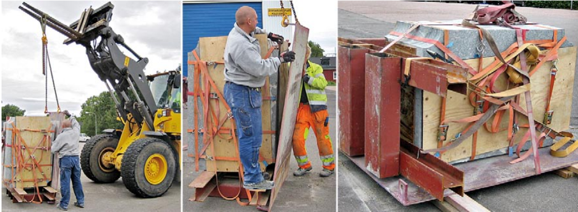
Figure 4-9. Gently tipping a block.
