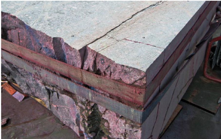
Figure 6-12. Block with block side with visible fracture traces.
