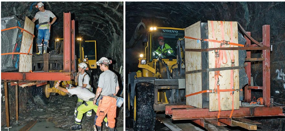
Figure 4-8. Removal of a block from the tunnel wall.
