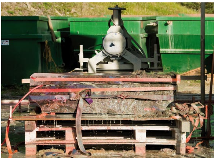
Figure 6-8. Block fixed at sawing place.
