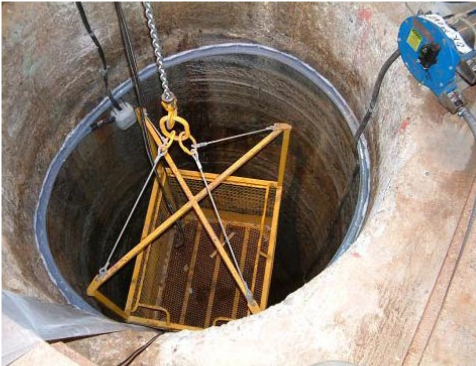
Figure 2-5. Deposition hole DA3147G01 with the circular drain and small plastic container (greyish).
