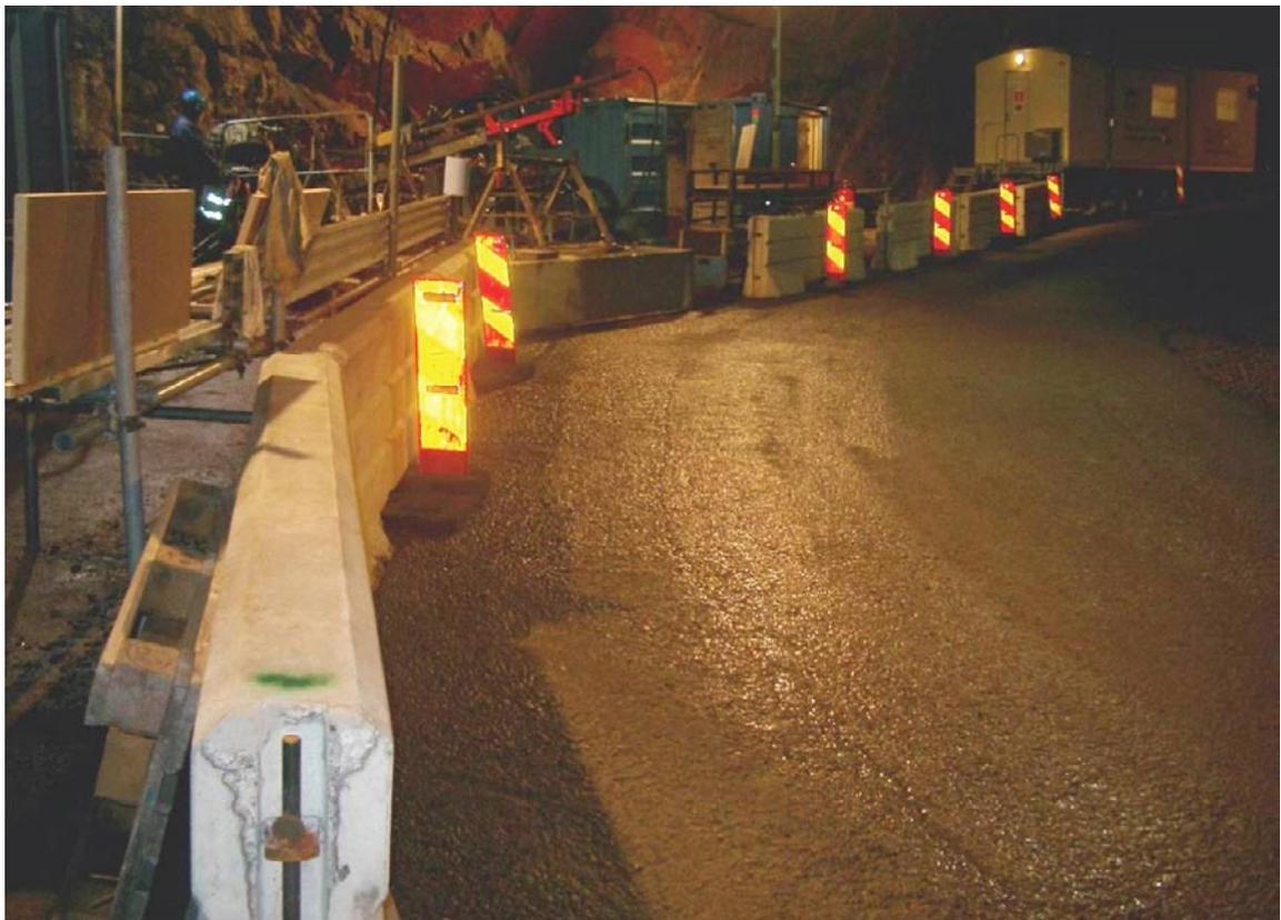
**Figure 5-4.** Specially designed cement blocks prohibited rolling vehicles from causing damage on personal or equipment on the drill site located in the curve at “Nedre Byggtunneln”.
