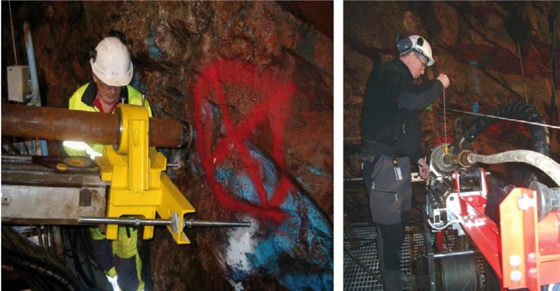
*Figure 5-12. Pre drilling was performed with the B116 dimension that gives a 116 mm borehole diameter and a 92 mm core diameter. The borehole direction was settled with two fixed points, one close to the borehole collaring and one backwards at the tunnel wall, after which a string was attached to the fixed points. By using a pendulum and a measuring tape, the drill rig could be adjusted accurately to the determined direction.*
