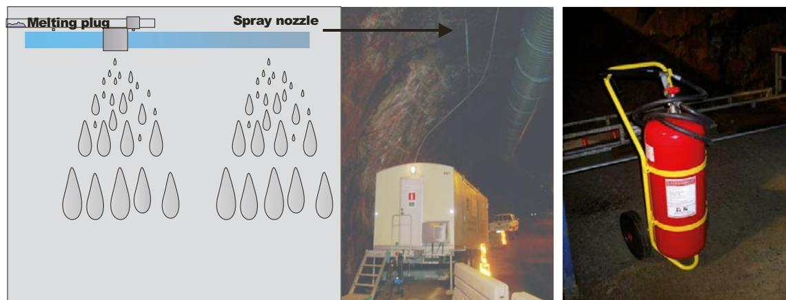
**Figure 5-2.** The extended fire prevention included a sprinkler mounted in the tunnel roof, covering most of the drill site. In addition, an extra fire-extinguisher (50 kg) was placed close to the drilling machine and the hydraulic unit.
