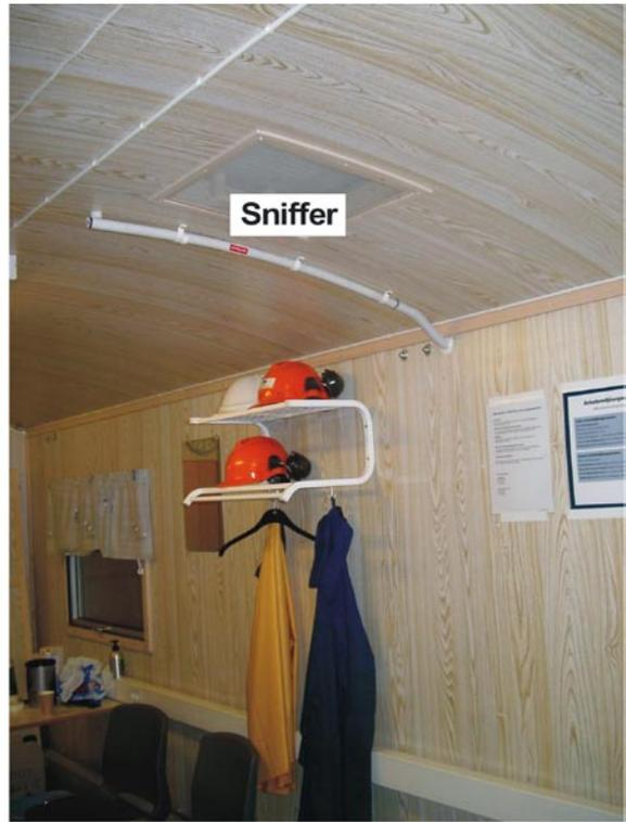
**Figure 5-3.** Left. Nitrogen was used for reduction of oxygen content in the flushing water tank. If nitrogen would leak out and cause a lack of oxygen in the air, the gas detector would alarm the drillers with a flashlight and a ringing bell. Right. In the personnel carriage a “sniffer” was installed in order to detect smoke from a fire. Therefore smoking is not allowed underground in the SFR-facility.
