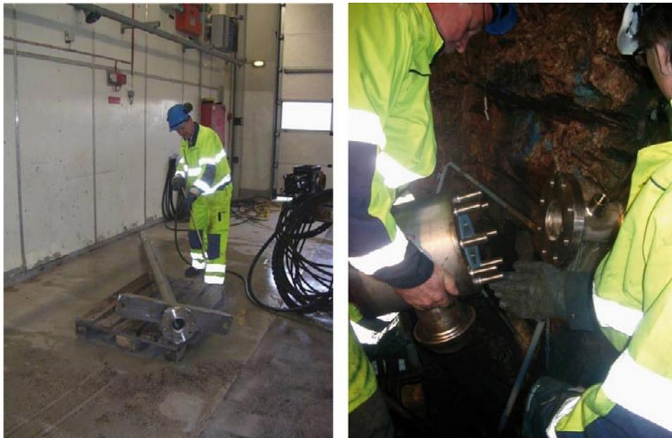
**Figure 5-11B.** Left. Cleaning with hot water on ground of the 3 m stainless steel casing. Right. Bolting of the casing to the rock wall after gap grouting in the pre-drilled borehole.
