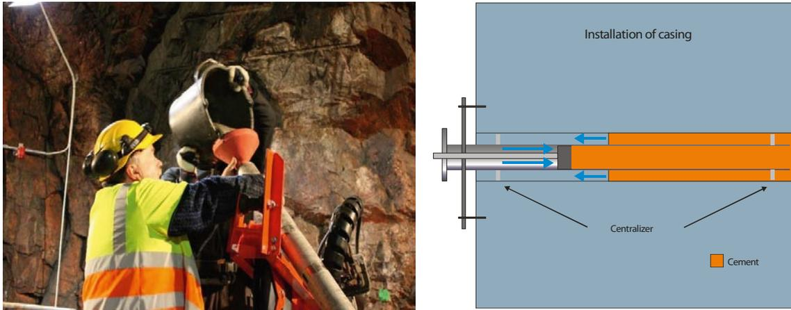
**Figure 5-13.** Grouting of casing. The casing was filled with cement, after which it was installed and centralized in the pre-drilled borehole. The cement grout was pressed backwards with a plug (a plastic piston), so that the cement was forced into the gap between the outside of the casing and the borehole wall.
