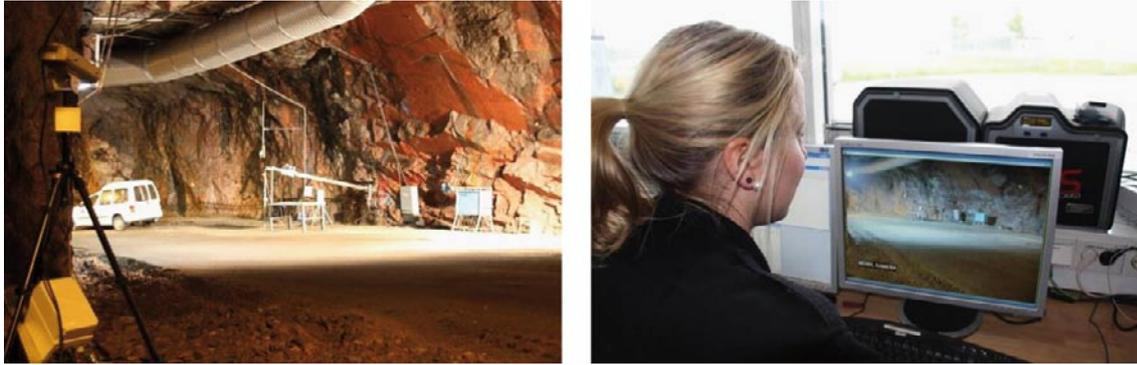
**Figure 5-5.** A video camera provided a perspicuous picture of the drill site and was connected to the SFR alarm system where the guard crew could supervise the ongoing work at the drill site.
