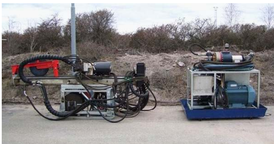
Figure 3-1. The Sandvik DE130 drilled boreholes KFR106.
