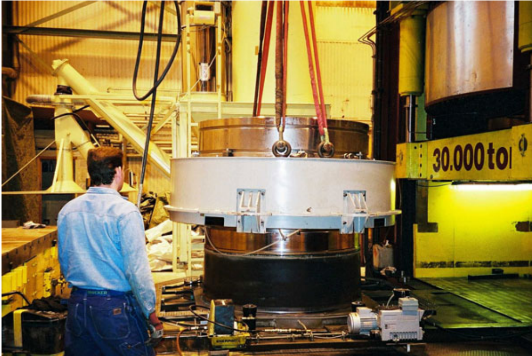
Figure 4-5. The bentonite block placed on the bottom plate while the form is removed.
