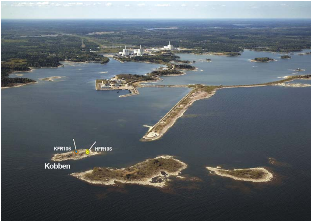
Figure 5-1. Overview of the surroundings at the Forsmark harbour area and SFR. The new drill sites for percussion borehole HFR106 and the cored borehole KFR106 are located on the islet “Kobben”.
