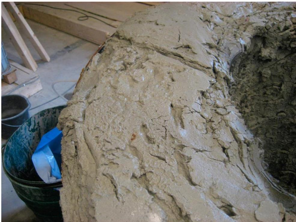
*Figure 4-33. Bentonite slurry on top of the ring.*
