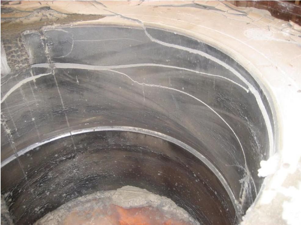
*Figure 4-35. Cracks on the inside of the uppermost ring.*
