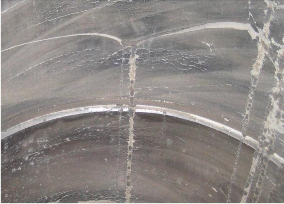
*Figure 4-36. Transport of material in a massive crack in the uppermost ring.*
