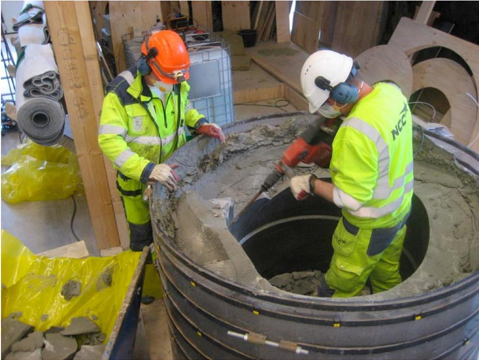
*Figure 4-25. Disassembling of the rings.*
