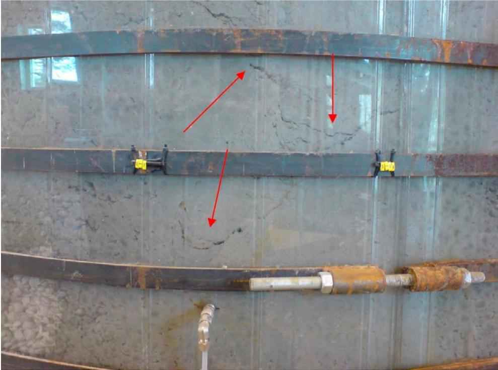
*Figure 4-17. Water pathways as a result of piping.*
