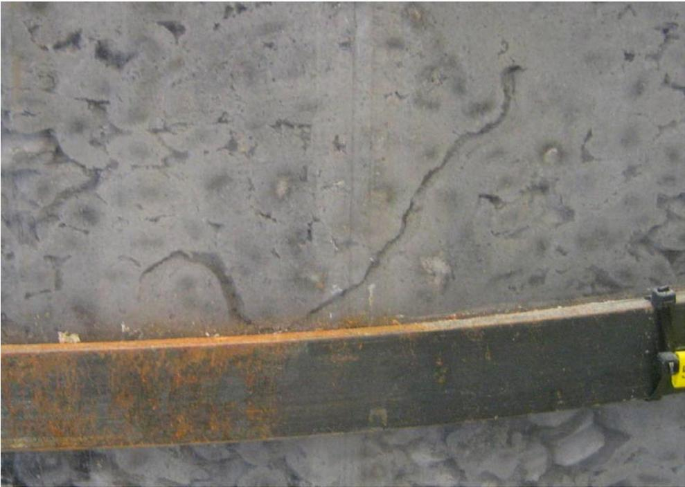
*Figure 4-18. Water pathway as a result of piping.*
