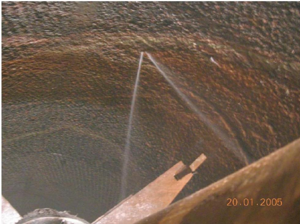
*Figure 2-2. Typical seepage pattern from a fracture zone /Bäckblom and Lindgren 2005/.*
