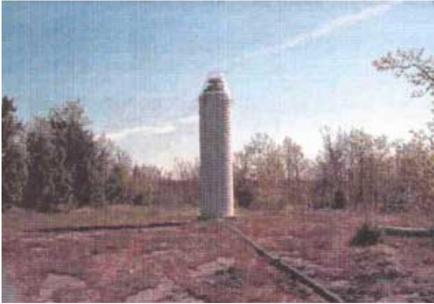
Figure 2.4. The SWEPOS station Oskarshamn with a choking antenna.
