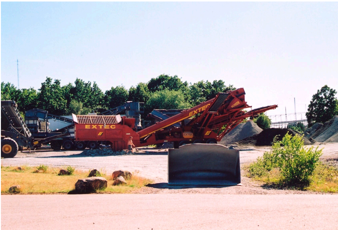
Figure 2-2. Photo of the crushing equipment.
