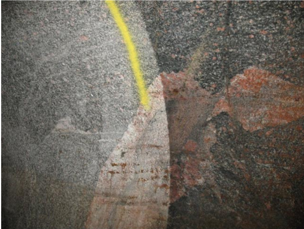
Figure 3-1. Picture showing a wet rock wall and a dry rock wall. This photo is showing that the performance test of the packers was performed perfectly and that the packers had an excellent sealing off effect.
