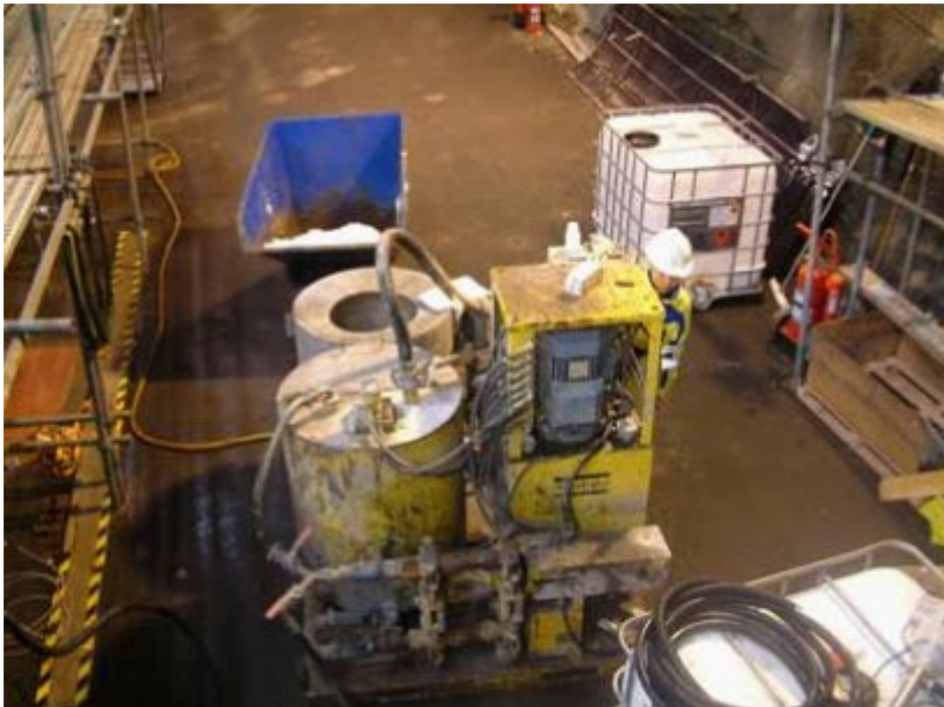
Figure 2-7. The Unigrout equipment used in November 2007.
