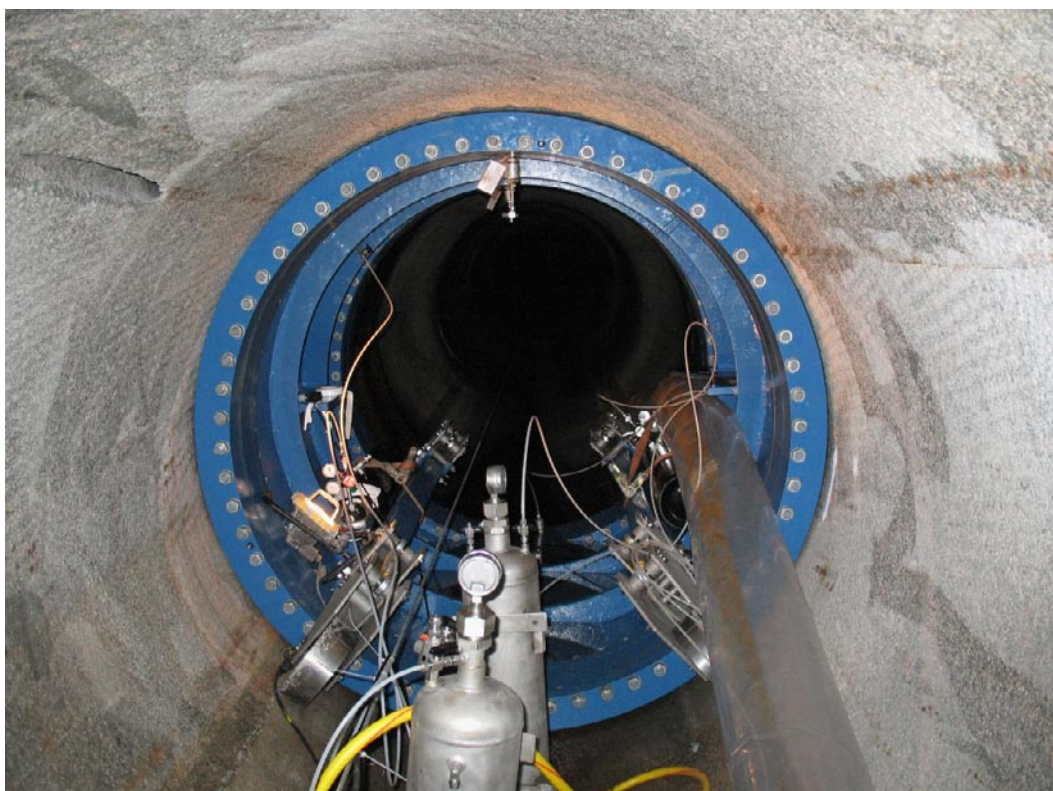
The Mega-Packer connected to the pressure tanks.
