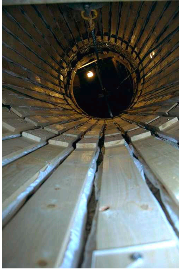
Figure 4-3 The deposition hole with applied diapers in DA3575G01.
