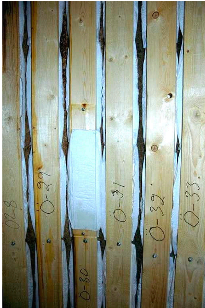
Figure 4-5 Reference diaper between plank and Plexiglas in DA3575G01.
