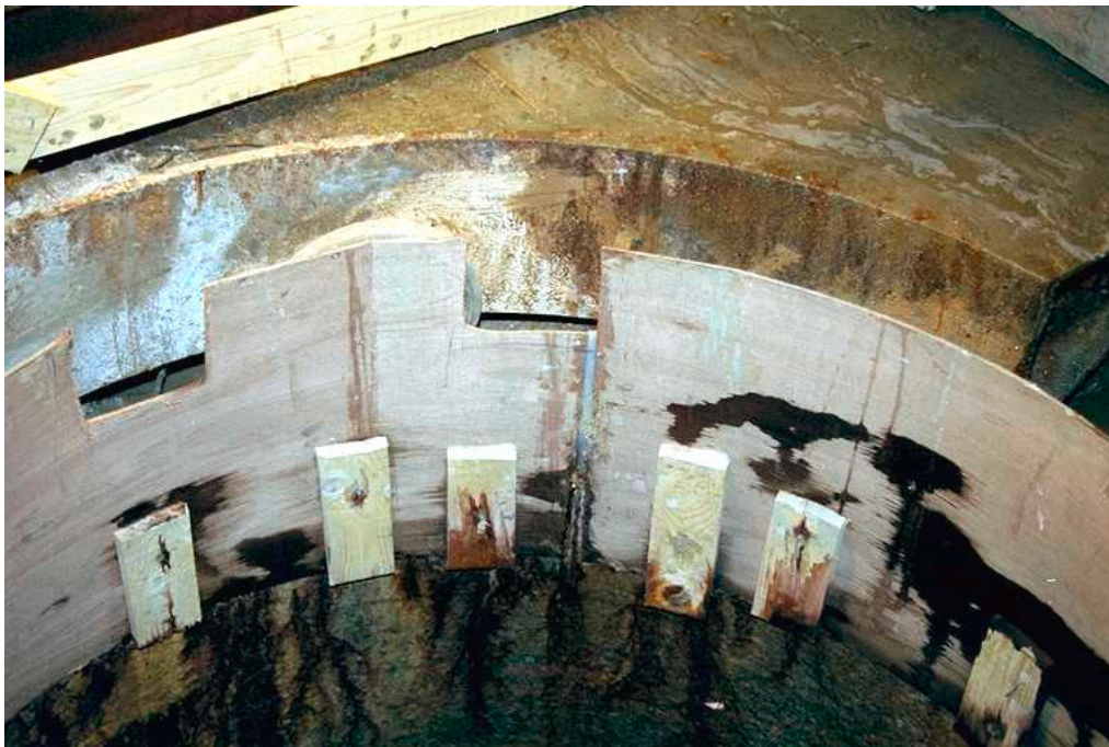
Figure 4-2 Upper part of hole before diapers were applied in DA3575G01.
