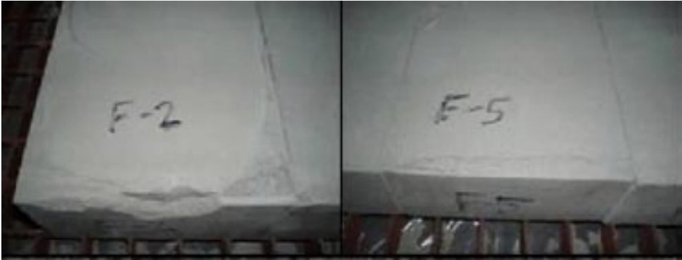
Figure A-3. Cracks in surface of lowermost blocks.
