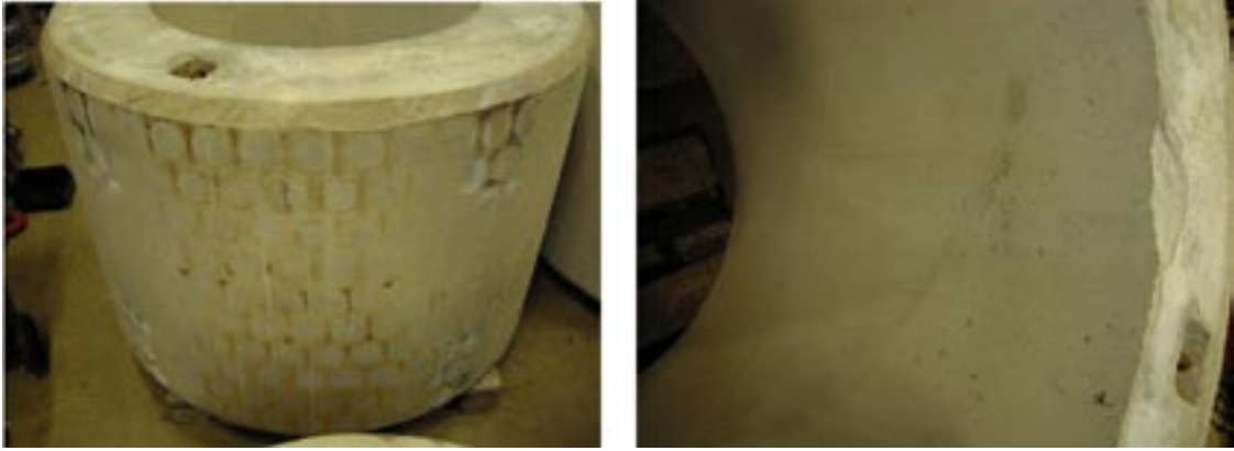
Figure 5-19. Examination of the concrete rings.
