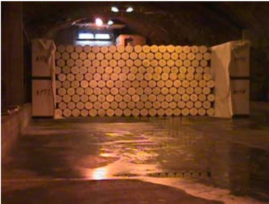
Figure 4-1. Inplacement of drums in 1BTF.
