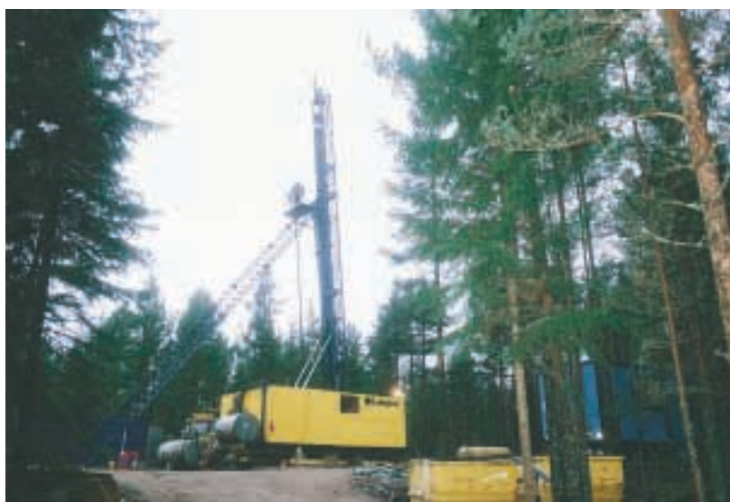
Figure 13-3. Core drilling on a prepared drilling site.
