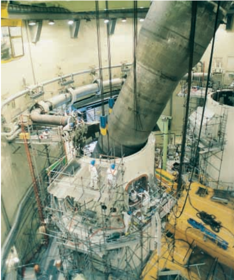
Figure 17-2. Replacement of steam generator in Ringhals.
