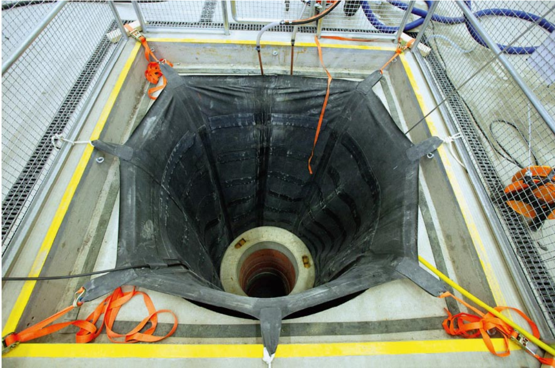
Figure 8-7. Installed buffer column.
