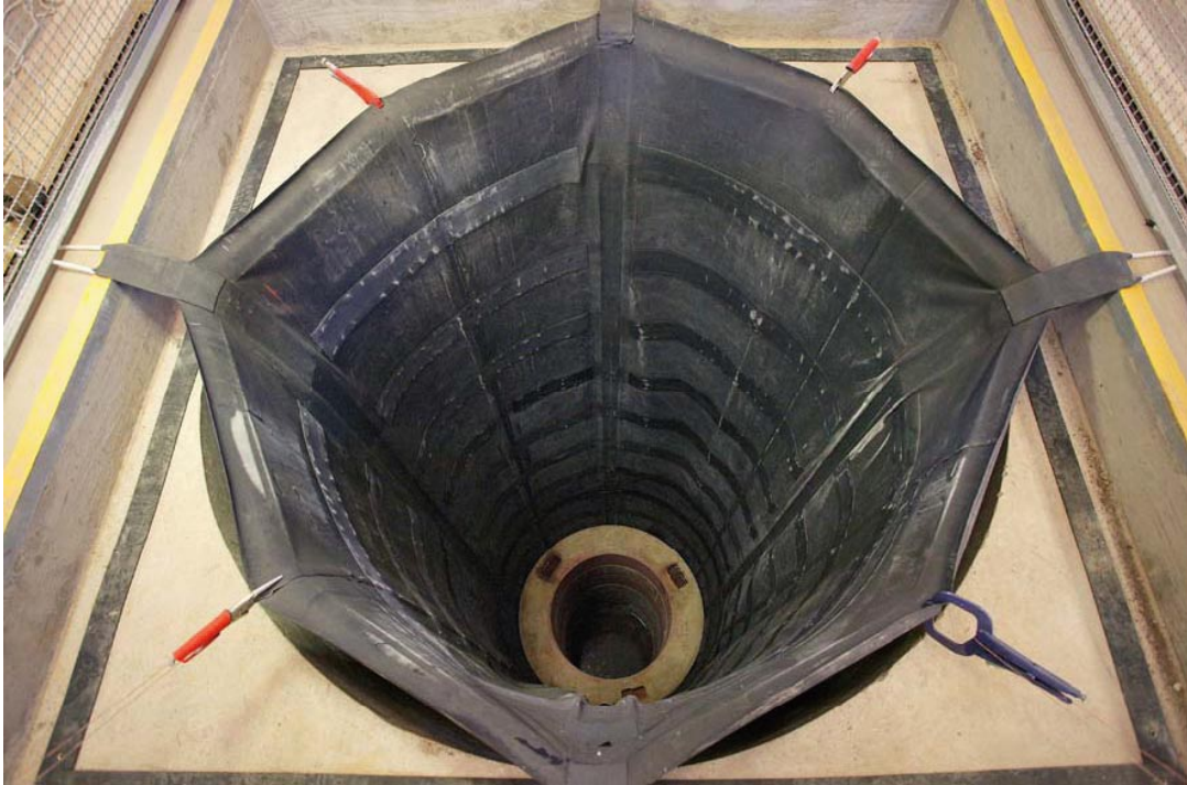
Figure 4-3. The buffer protection sheet with supporting rings mounted in a deposition hole.
