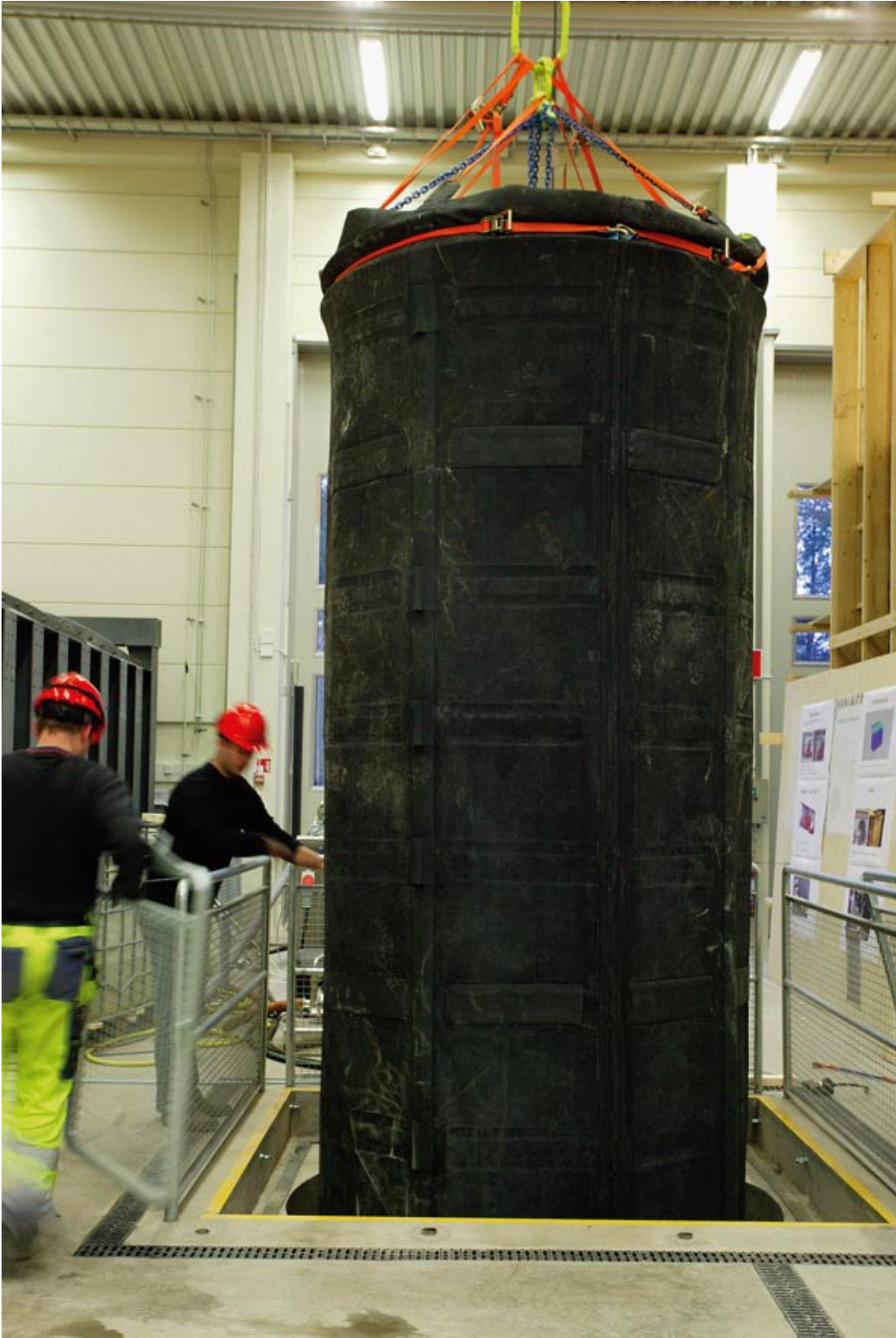
Figure 8-6. Installation of the buffer protection sheet.
