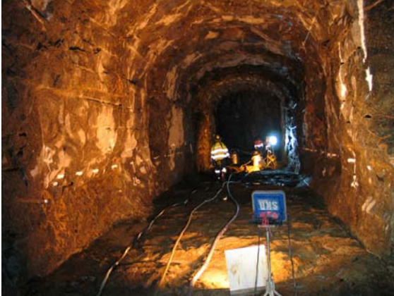
Preparations before mapping of the Tass-tunnel (photo: Oskar Sigurdsson)
