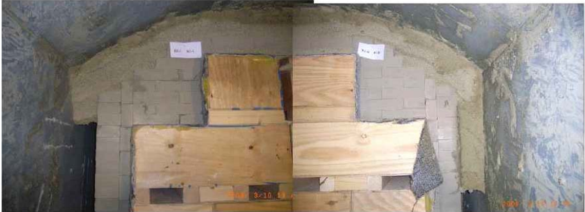
Figure 6-6. Wetting along crown of Assembly 3 (Tests 5, 6). (Note dry (empty regions along walls) and wetting (darker regions) along crown.
