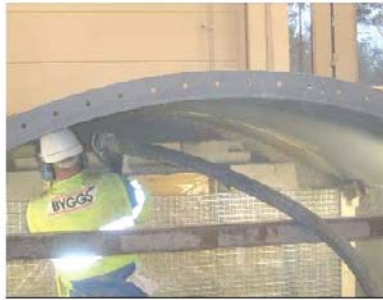
Blowing pellets into crown
