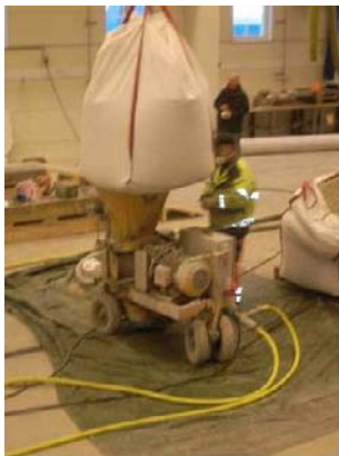
Supplying pellets to shotcrete machine
