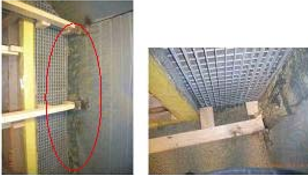
Figure 6-16. Face of Test 12 showing damp surface exiting pellet fill.
