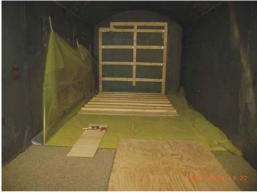
Pellets Installed on Floor
