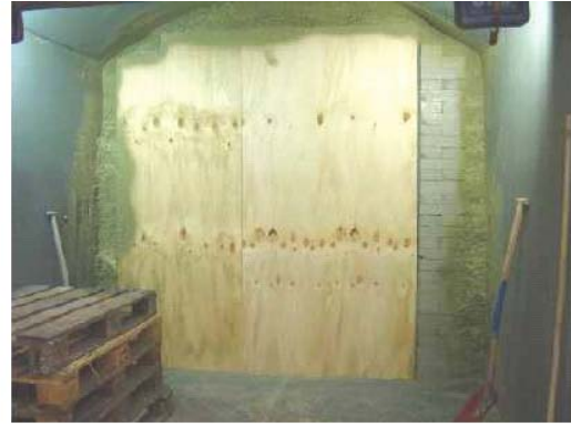
Setup following clay pellet installation
