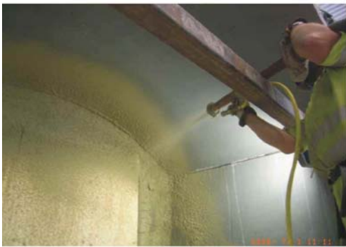
Blowing Wet Pellets at Downstream Face
