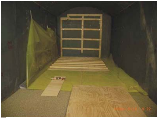
Pellets Installed on Floor
