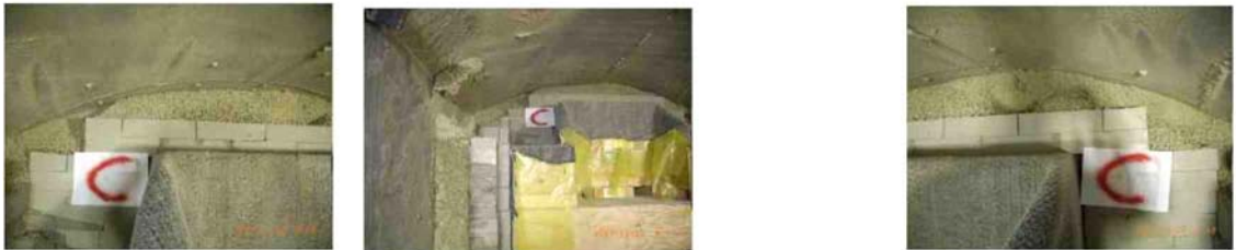
Central portion of Test 1 and Test 2 showing dry crown region
