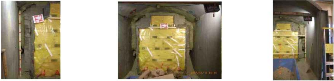
Front face of Test 1 and Test 2 once surface layer removed
