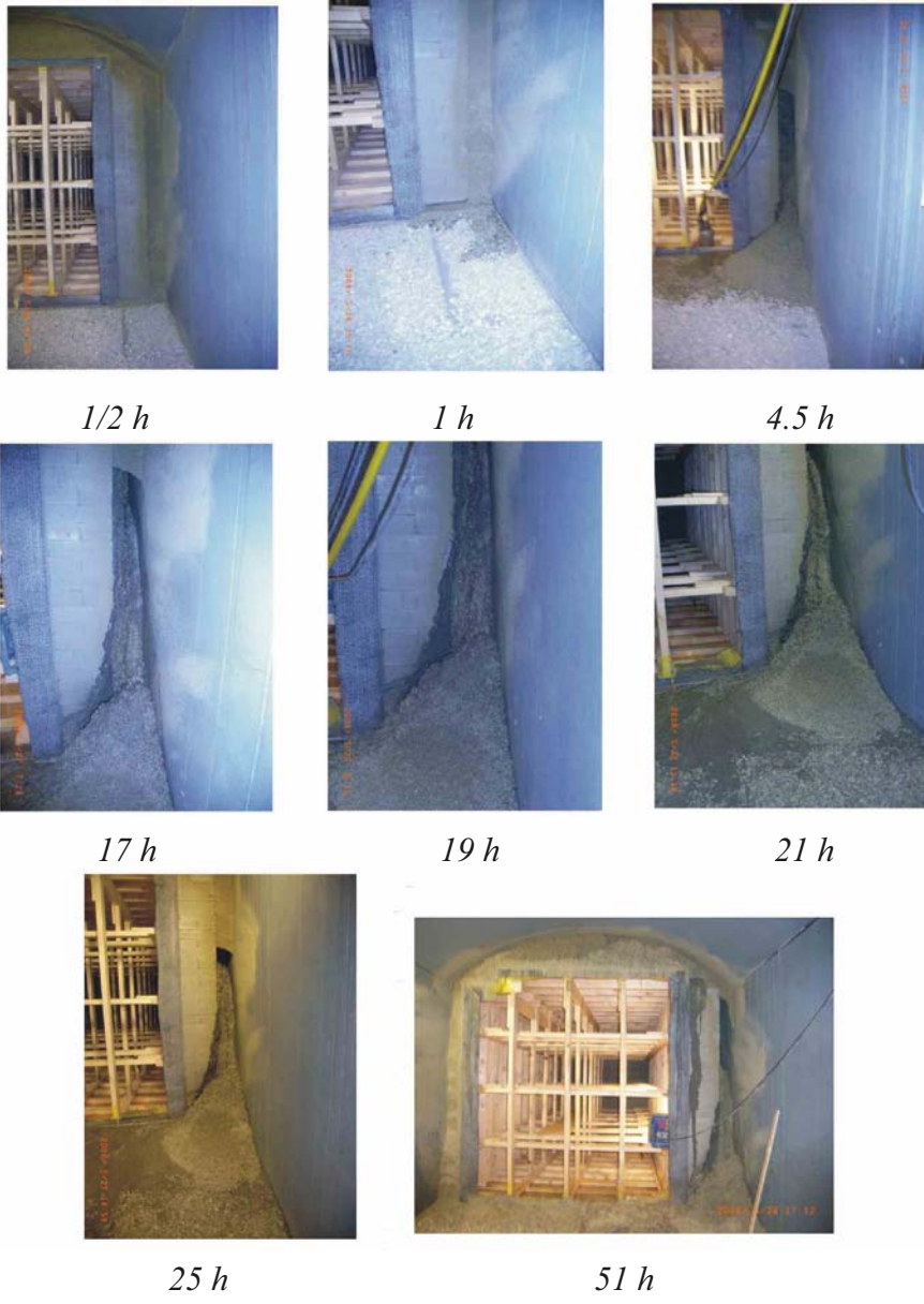
Figure 6-24. Ongoing erosion at inflow rate of 2.5 l/min.
