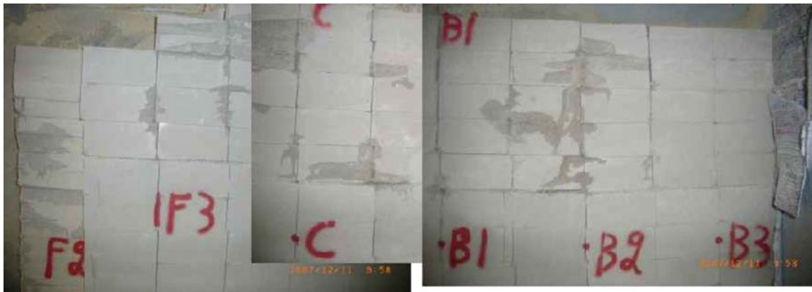
Figure A-3. Movement of water along block joints near top of Test 1. (view from front (F) to back (B)).
