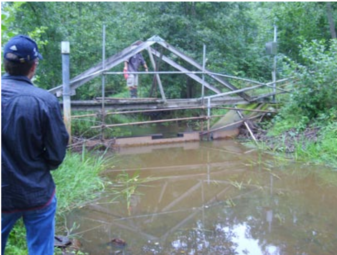
Figure 2-45. The two rectangular notches at PSM000364. The discharge is calculated in the same manner as for a natural critical section.
