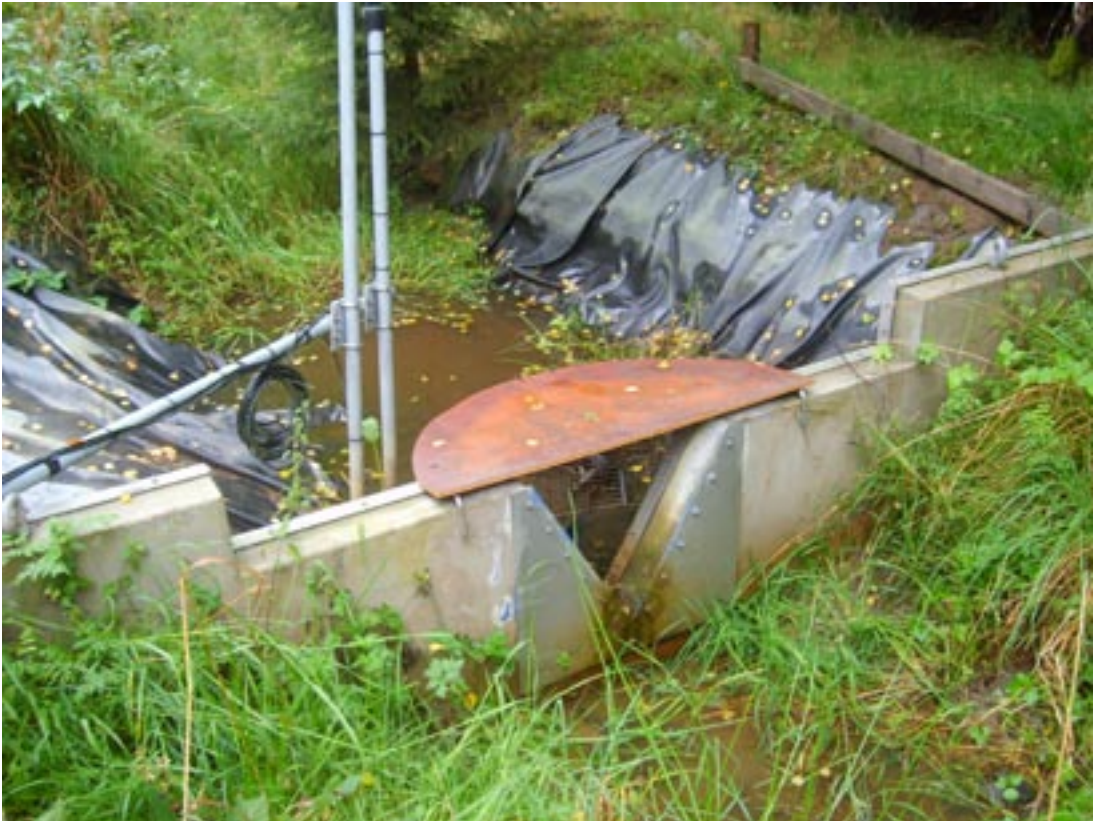
Figure 2-42. V-notch weir at gauging station PSM000347.
