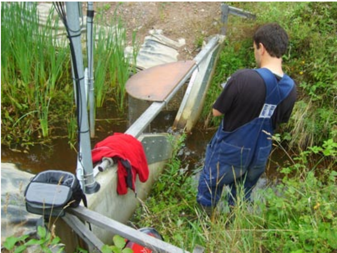
Figure 2-47. V-notch weir at gauging station PSM000365.
