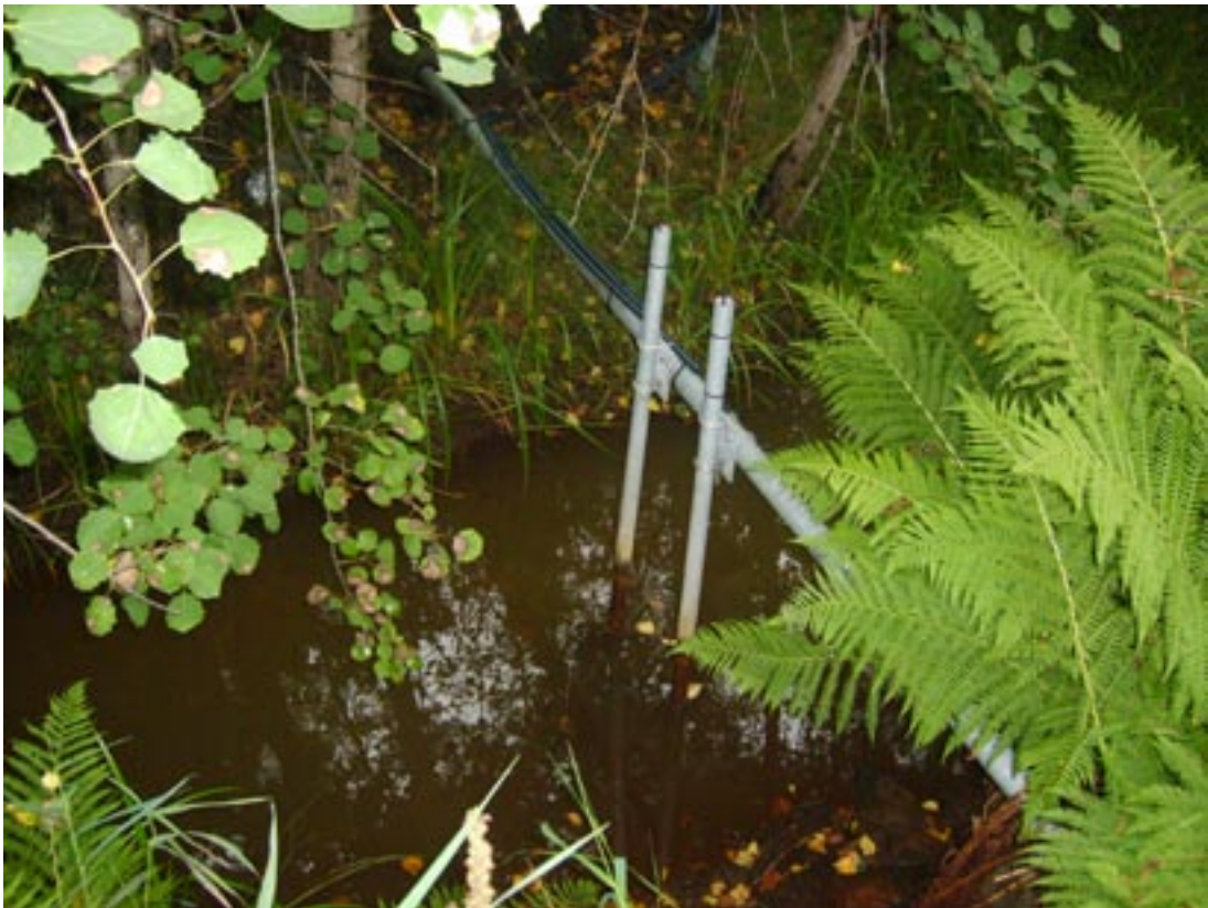
Figure 2-44. Water-level instrumentation at gauging station PSM000353. The natural critical section is likely a road culvert downstream from this site.
