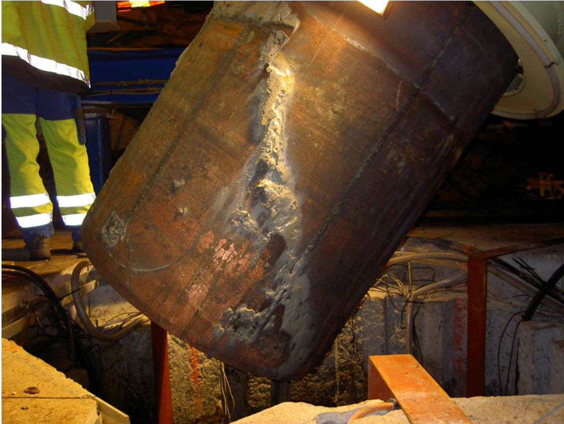
Figure 24. Some remaining bentonite on the canister. The uneven levels of buffer around the canister after the disintegration forced the disintegration to be stopped before the entire canister was freed from the buffer. Despite this it was no problem to lift the canister from the deposit hole.
