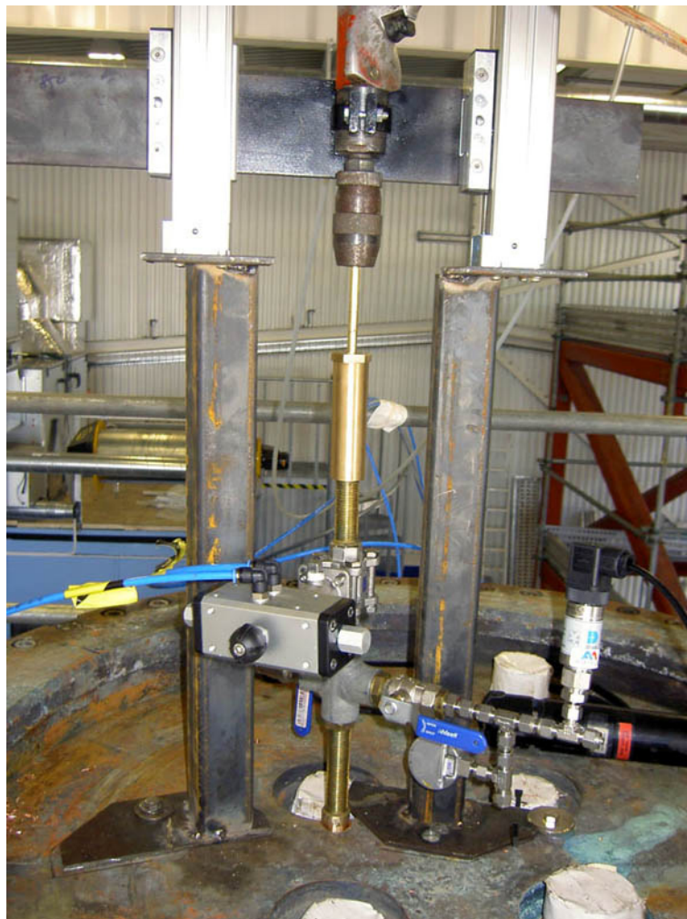
Figure 19. Mounting of the valve with the hot tap equipment. The picture is taken just prior the process of puncturing the canister.
