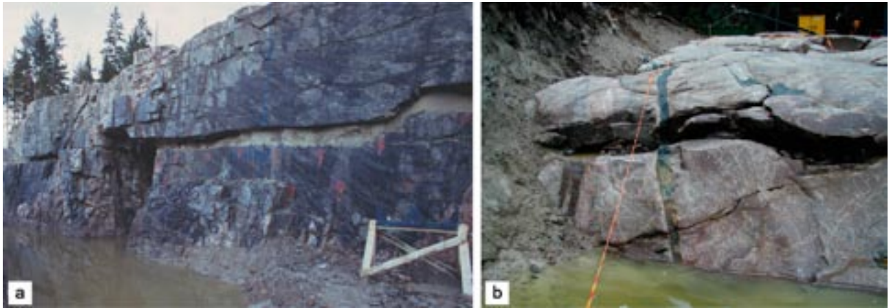
Figure 2-23. Subhorizontal and gently dipping fractures close to the current ground surface at Forsmark. a) Subhorizontal fracture filled with glacial sediment inferred to be a sheet joint formed in connection with release of stress close to the ground surface. Excavation for unit 3 at the nuclear power plant /after Carlsson 1979/. b) Gently dipping fracture with wide aperture at drill site 5. The impressive aperture along this fracture is also inferred to have formed in connection with the release of stress close to the ground surface. Several fractures with this orientation at drill site 5 are filled with glacial sediment. See also section 3.4.2.
