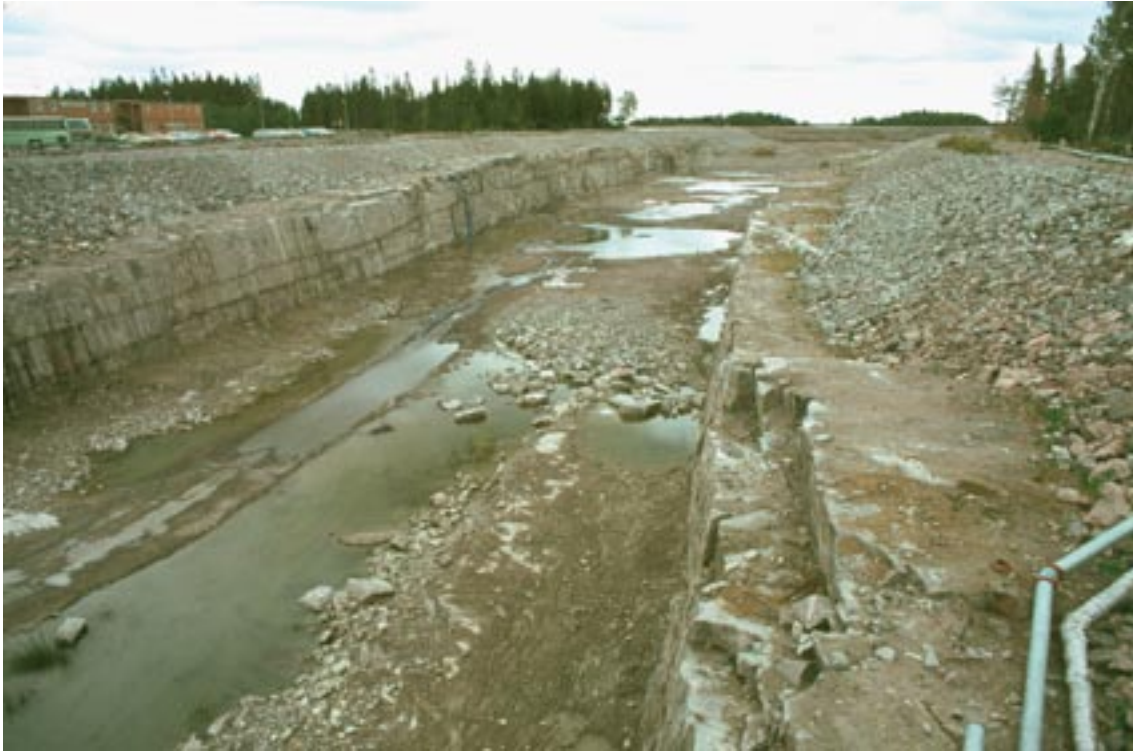
Figure 3-22. Picture from the construction of the 13 m deep and more than one kilometre long canal between the Baltic Sea and the nuclear power reactors. Horizontal fractures/sheet joints are encountered along the entire excavation. There are several “horizons” of extensive sheet joints on top of each other. The picture is taken from the southern side of the canal where the bridge crosses the canal between drill sites 7 and 8, see Figure B-1 in Appendix B.
