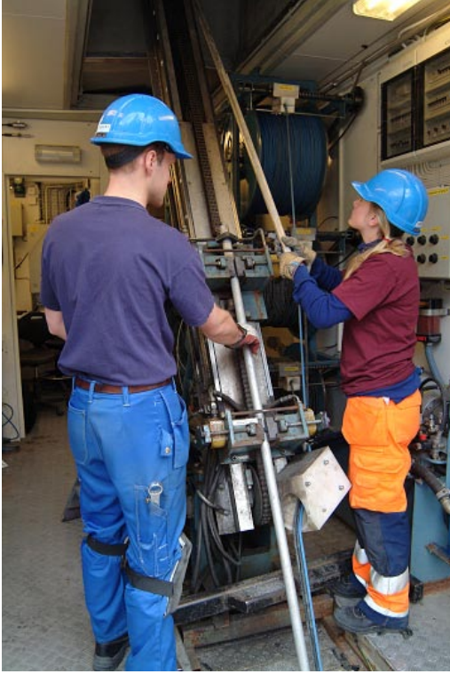
Figure 4-3. Lowering of aluminium-pipes into the borehole during pumping with PSS3.
