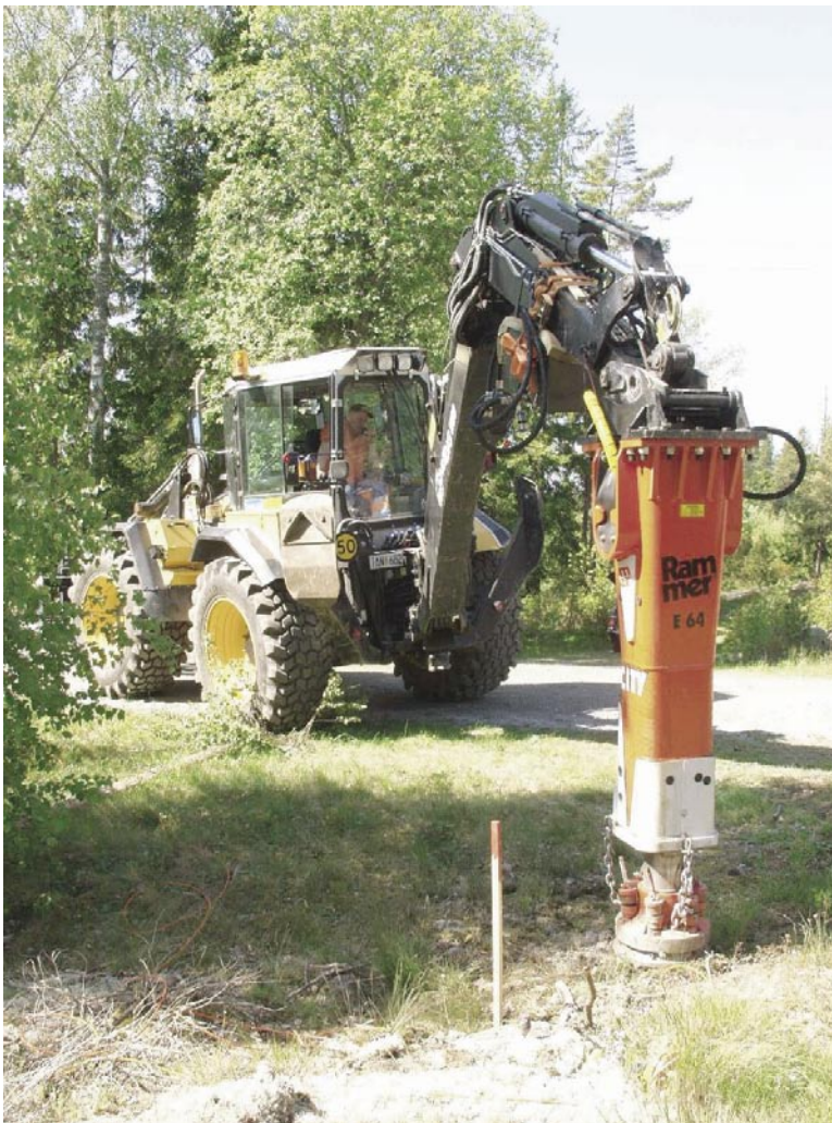
Figure 5-1. Hydraulic hammer and tractor used for the VIBSIST test.
