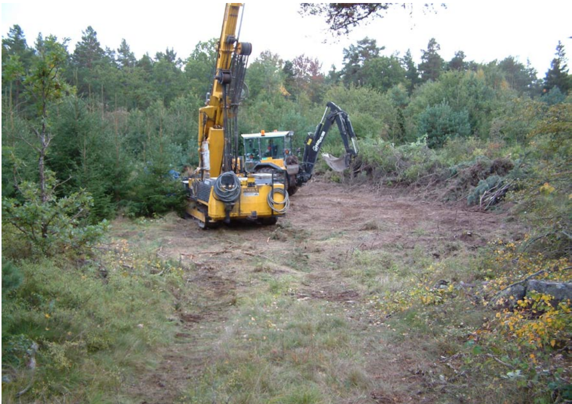
Figure 2-1. Establishing the percussion drill rig at the drill site.
