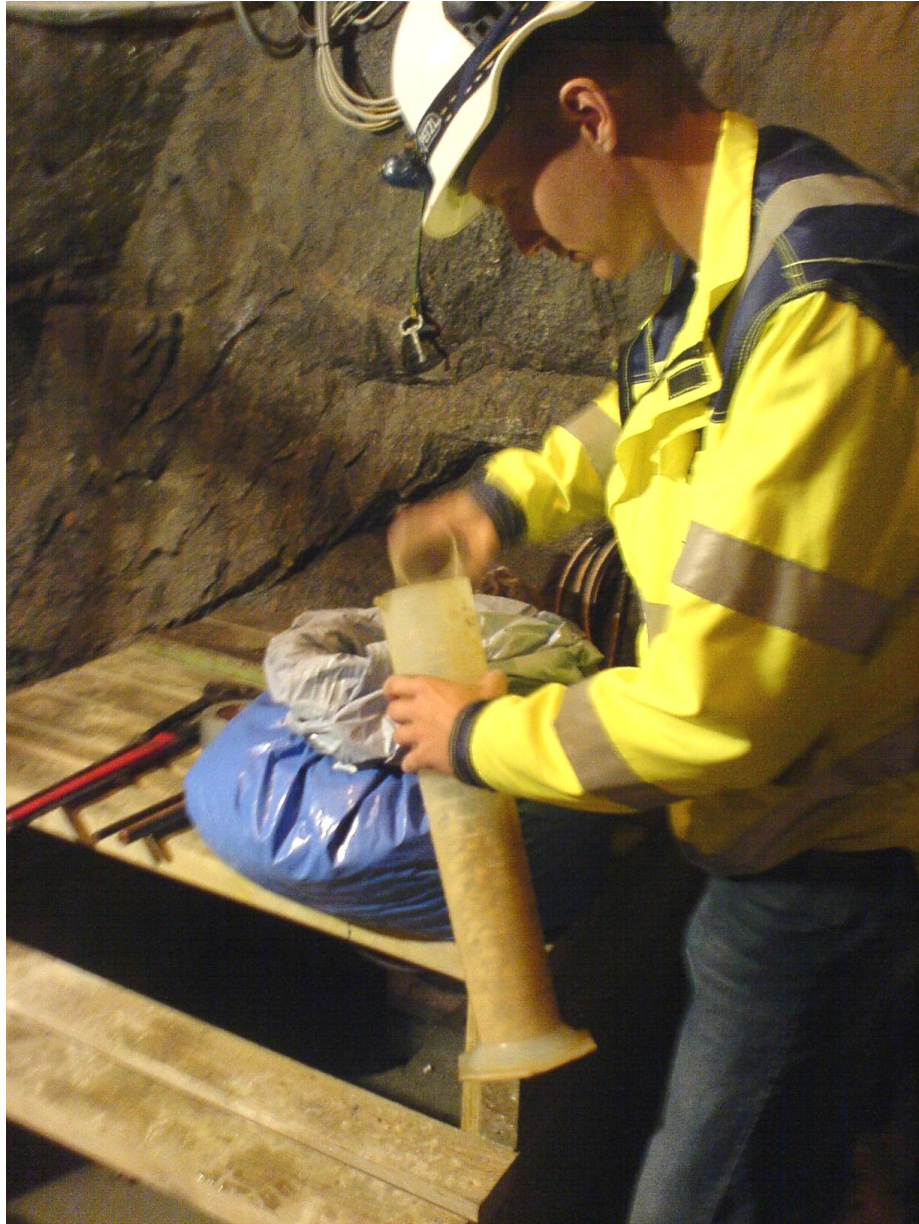
Figure 4-1. Pouring pellets in cylinder with known volume for subsequent filling of Hole D.
