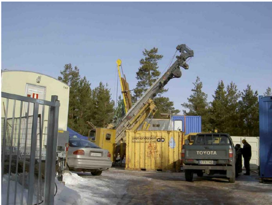
Figure 3-2. The drill site at KLX11A.
