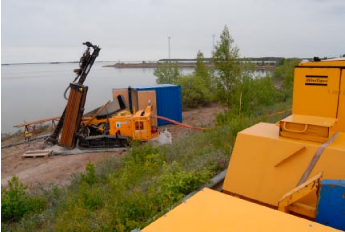
Figure 3-2. The Nemek 407 RE drilling machine at drill site DS11.
