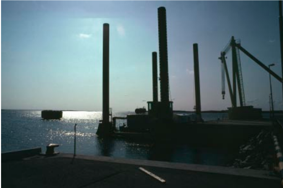
Figure 5-1. Offshore platforms were used for the exploratory core drillings for the SFR.
