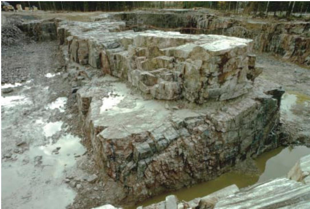
Figure 3-8. Photograph of shaft walls of the storage basin for industrial water showing continuous horizontal fractures containing filling material of sediments. The length of the shaft is approximately 100 m. Photo G Hansson/N.
