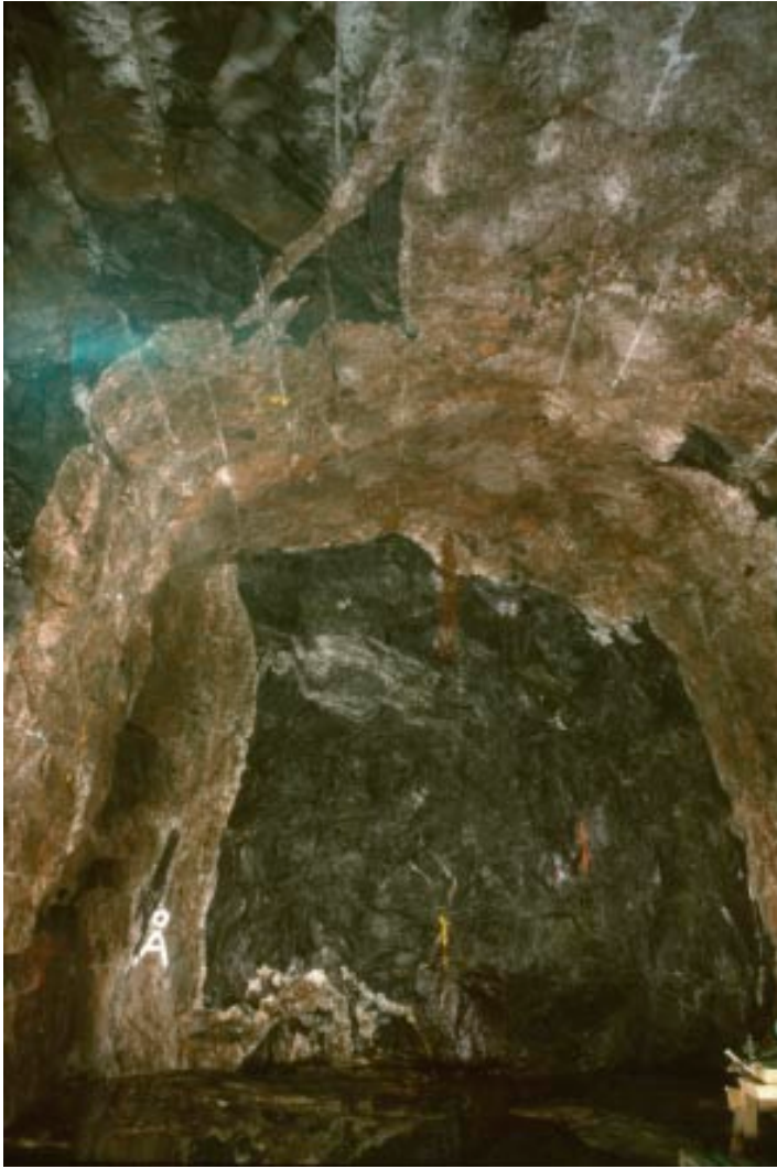
Figure 7-4. Pegmatite dykes at the face of the Forsmark tunnel. Host rock is mafic rocks.
