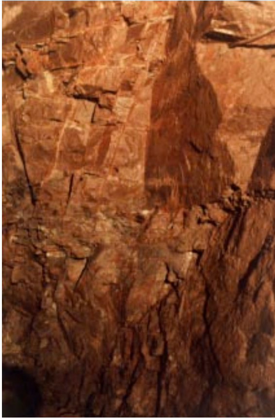
Figure 7-6a (left). Gentle dipping fractures within the deformation zone H2 under the silo of SFR. A section with relatively low fracture frequency.
