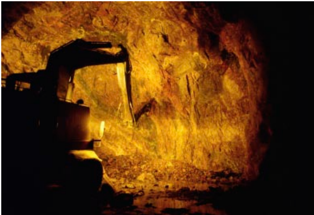
Figure 6-1. Mechanized scaling with a hydraulic hammer in the SFR tunnels.
