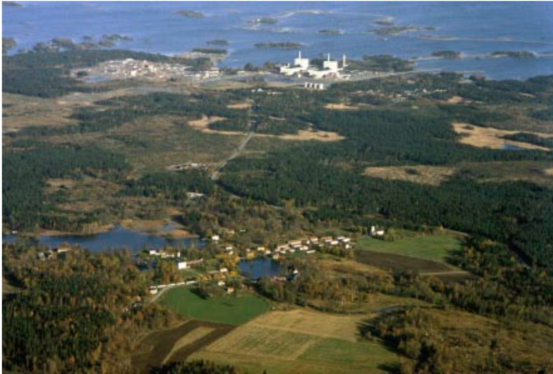
Figure 3-4. Aerial photo from 1980 showing the Forsmark construction area (Forsmark 3 is under construction); in the foreground, Forsmarks Bruk. Photo G Hansson/N.
