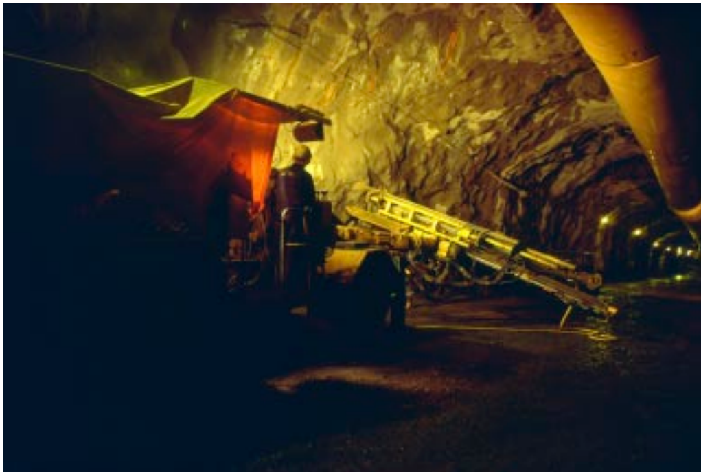
Figure 6-2. Mechanized rock bolting equipment used for bolting operations in the SFR.
