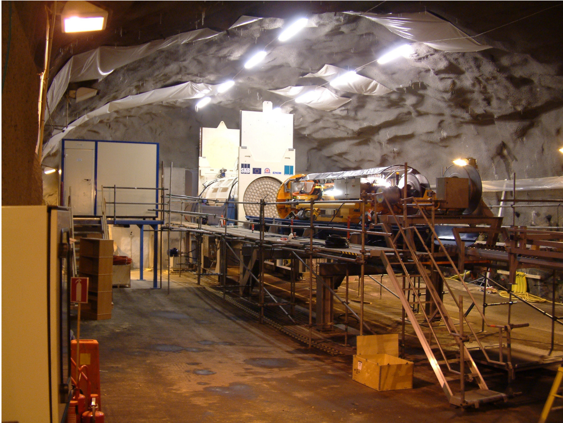
Figure 4-7 The deposition equipment in the niche at -220 m level at Äspö HRL.
