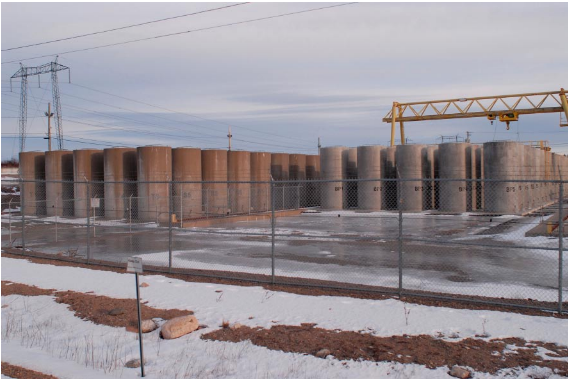
Figur 2-2. Utomhuslagring vid NB Power Nuclear – Point Lepreau Generating Station, New Brunswick Kanada – "Solid Radioactive Waste Management Facility – Dry Fuel Canisters". Källa: NBPower Nuclear.
