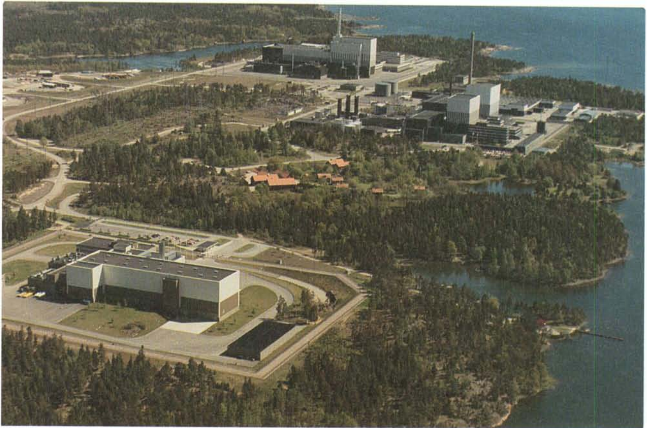
Figure 2-1. The Oskarshamn Nuclear Site. CLAB in the foreground.
