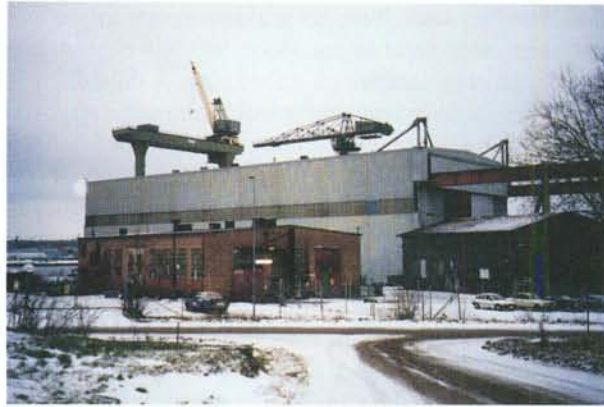
Figure 6.3. Canister Laboratory at the shipyard in the city of Oskarshamn.
